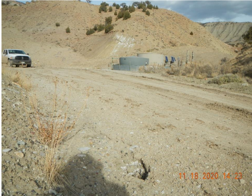
Channeling on edge of access road near entrance of location.
