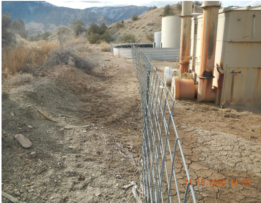
Sediment movement behind separators.
