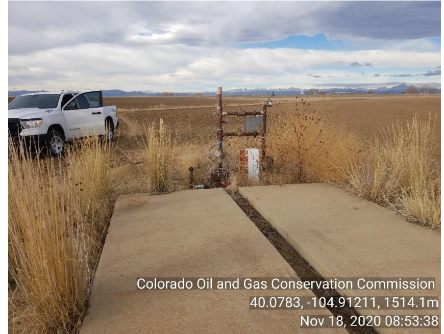
Photo 2 Sign is not posted properly and contact number has peeled off. Unused equipment Cement base is not being used.
