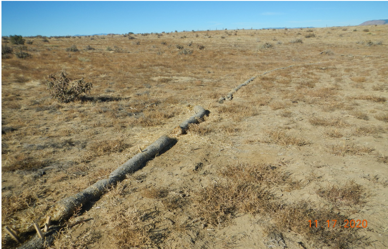
Photo 6. The wattles around the perimeter of the location are displaced and not maintained.
