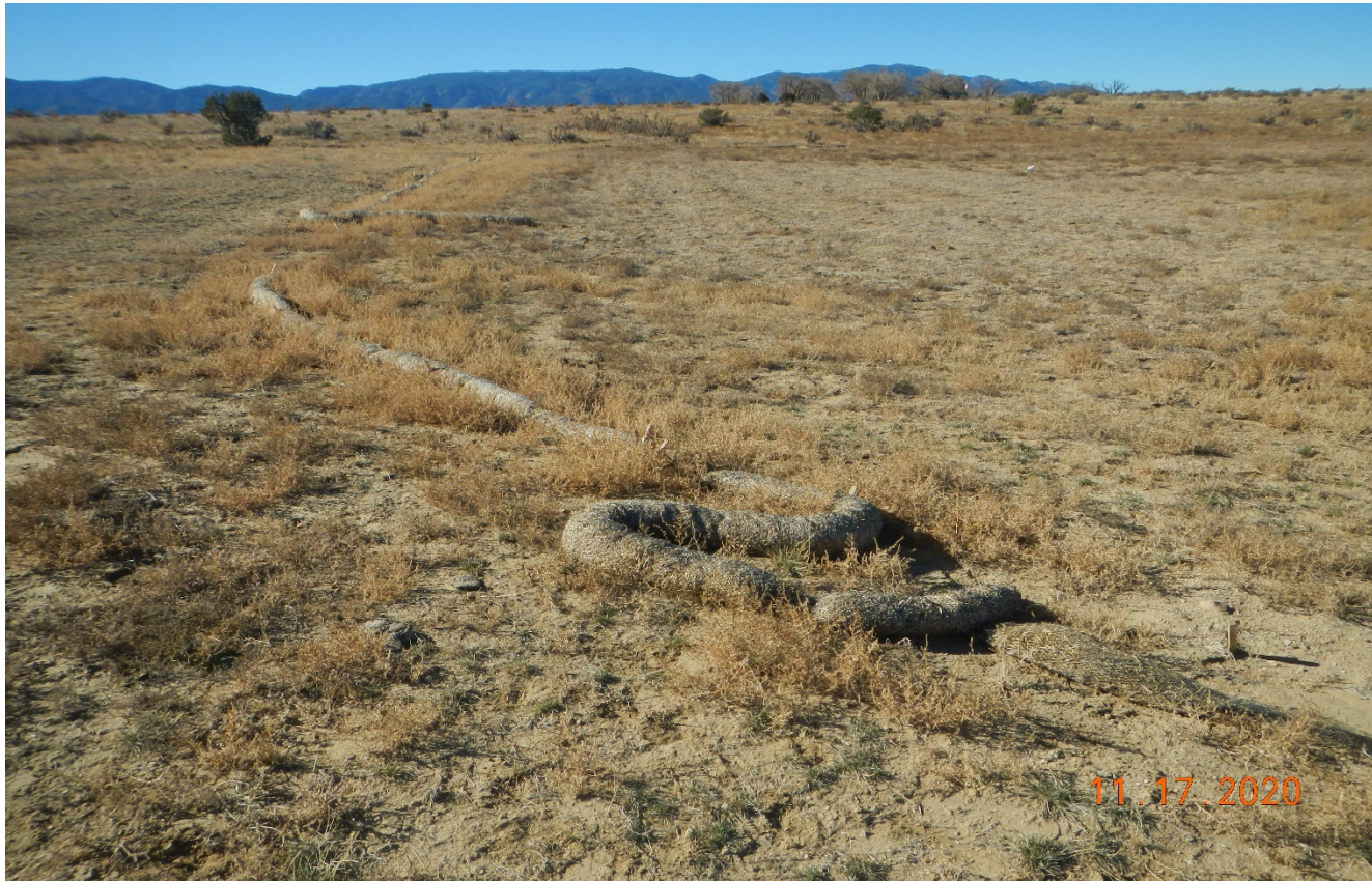
Photo 3. The wattles around the perimeter of the location are displaced and not maintained.
