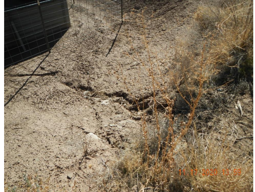
Rill of soft cut slope around tank battery.
