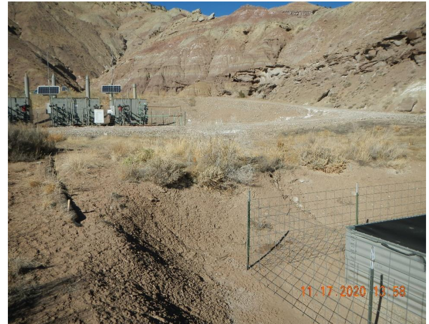
Riling of soft cut slope around tank battery.
