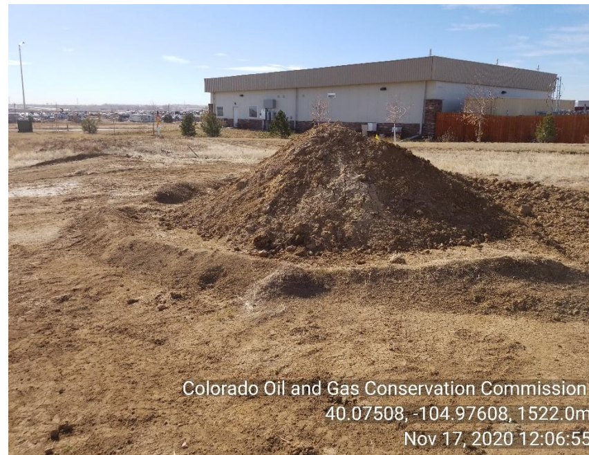
Photo 4 inadequate berm around oily material from spill.
