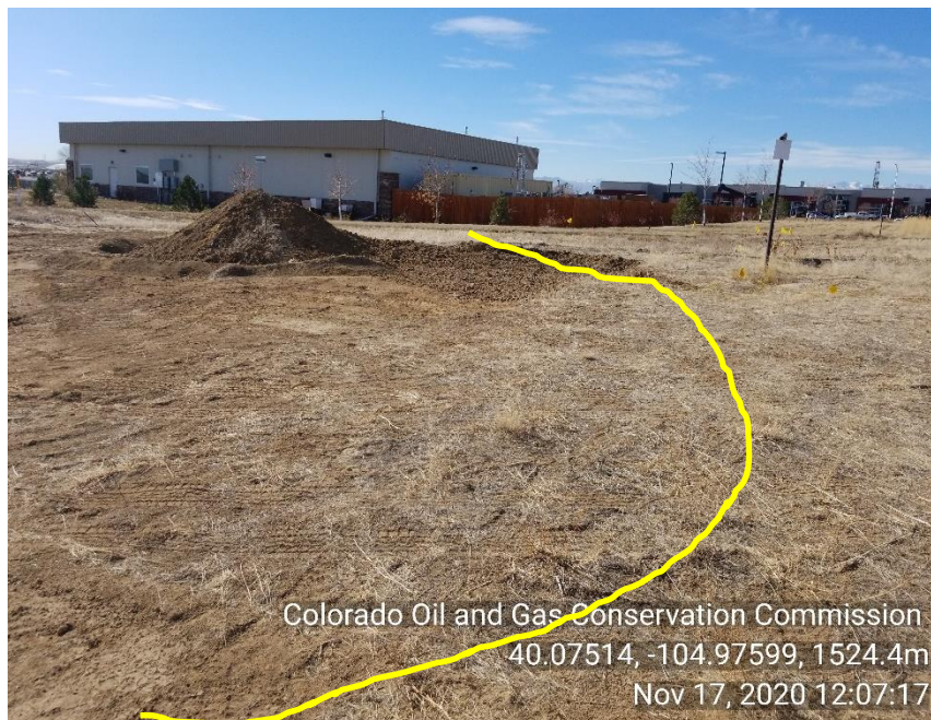
Photo 5 1 Disturbed area from spill remediation. No BMP's in place
