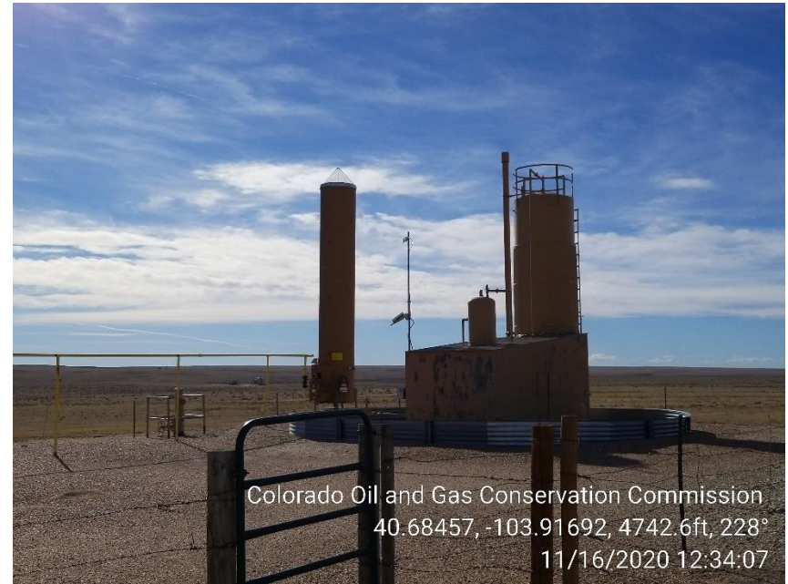
Photo 4 – Heater Treater, ECD
