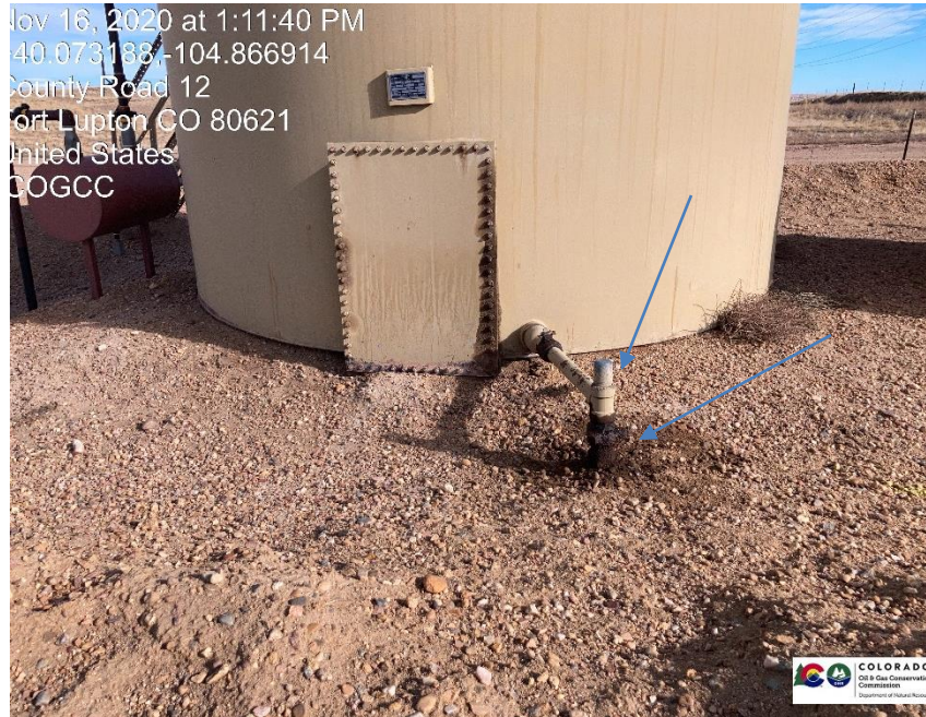
Pic 9 mechanical issue / stained soil
