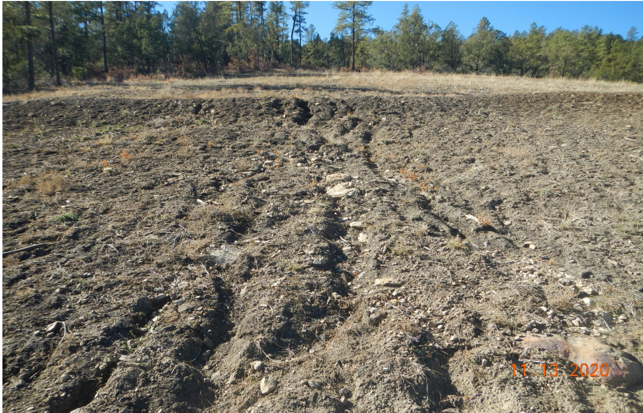
Photo 6. Facing west toward the location. The berms along the slope have failed causing stormwater to concentrate down areas of the location.
