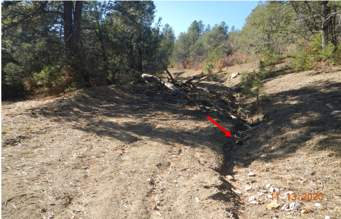
Photo 1. Facing southwest the beginning of the access road. The access road has not been recontoured and reclaimed. There are signs of erosion occurring down the road.
