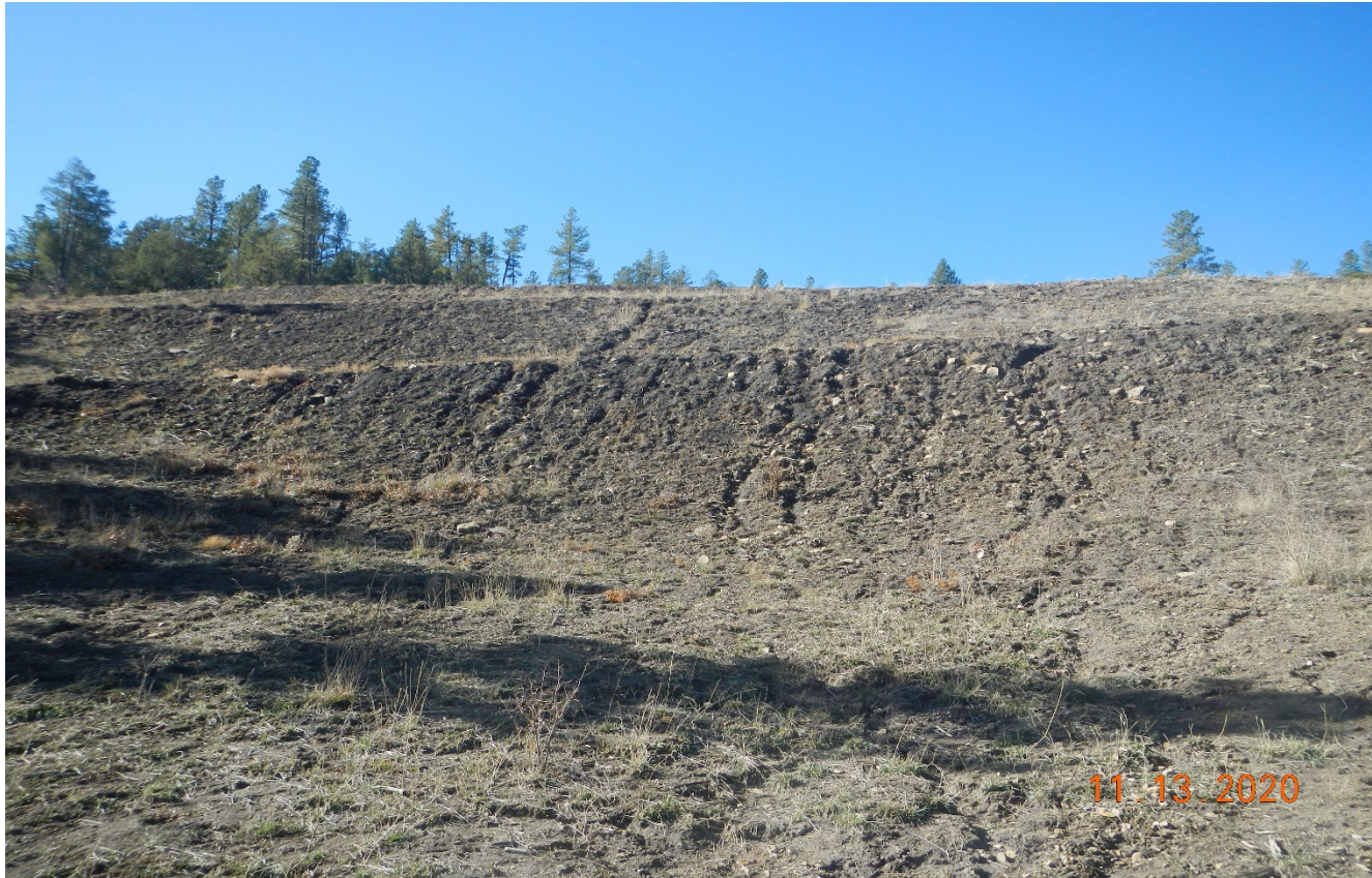
Photo 7. Facing west toward the location standing at the bottom of the slope. It appears the terracing performed has increased the degree of slope. The location appears rounded and should have been sloped down and tapered to reduce the slope.
