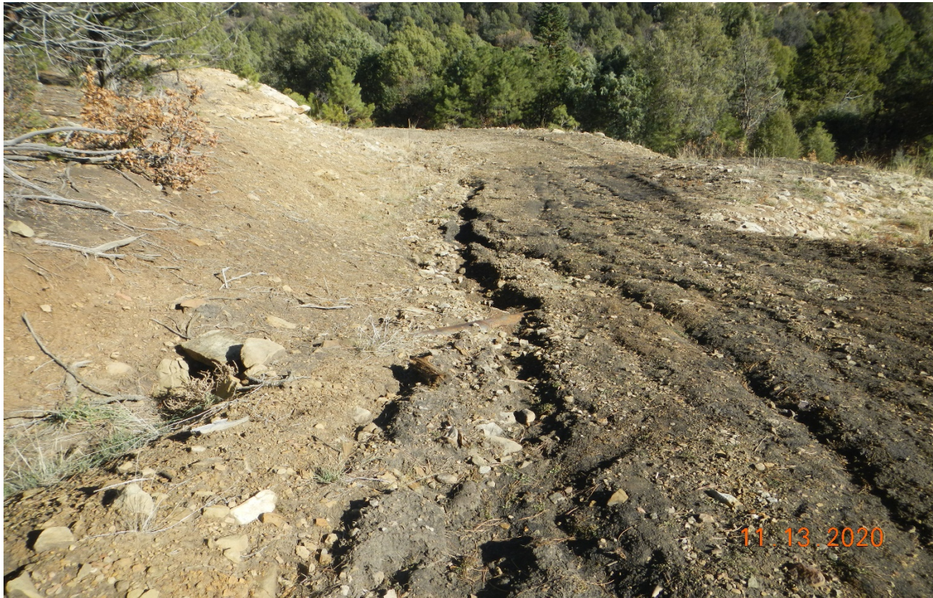
Photo 3. Facing northeast toward the access road. The culvert remains and erosion is occurring down the road.
