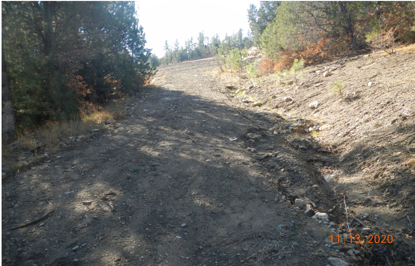
Photo 2. Facing south. The access road has not been recontoured and reclaimed.
