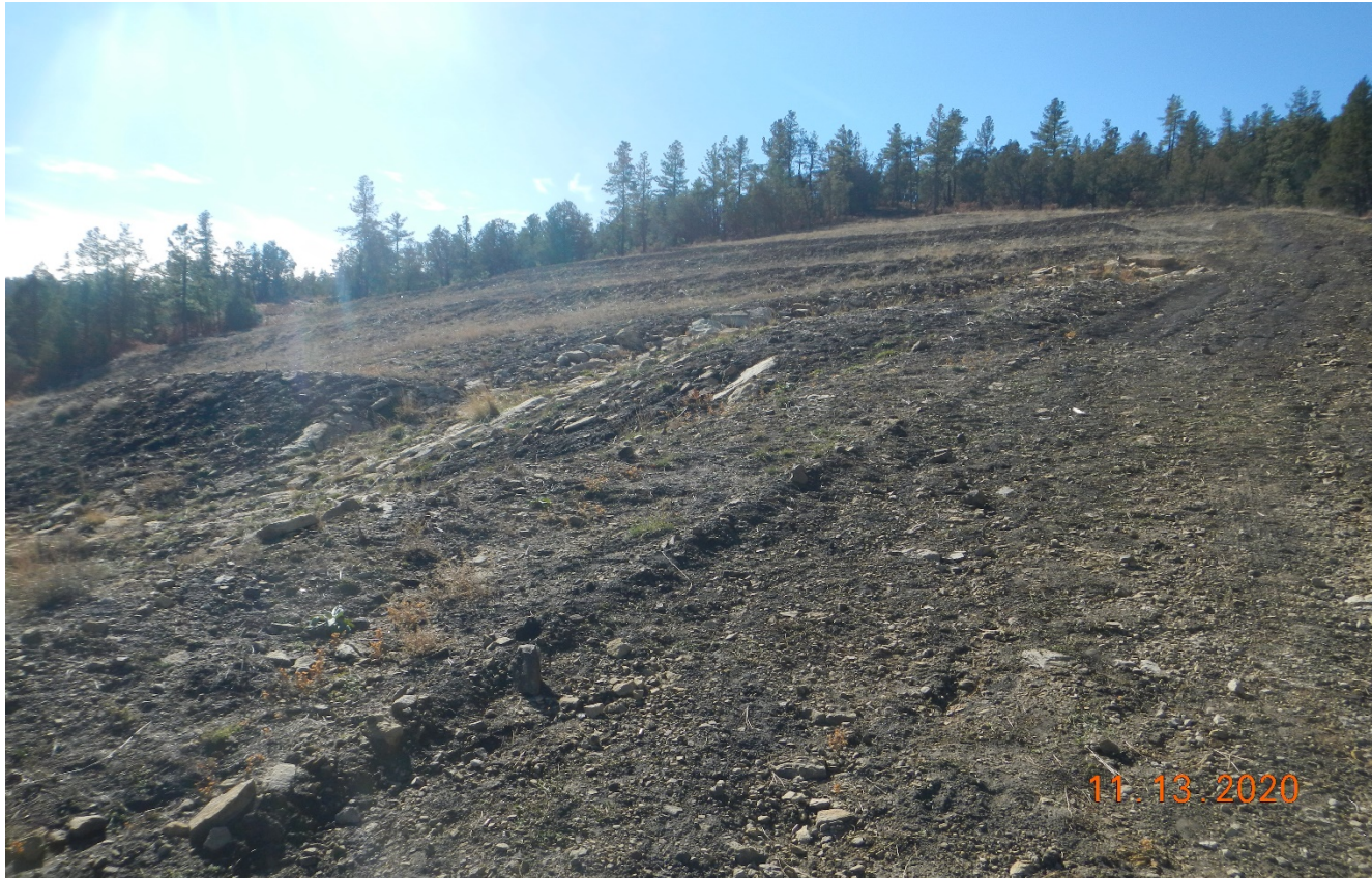
Photo 4. Facing southwest toward the location. The location has been recontoured however it has been terraced which does not match the original contours of the terrain.
