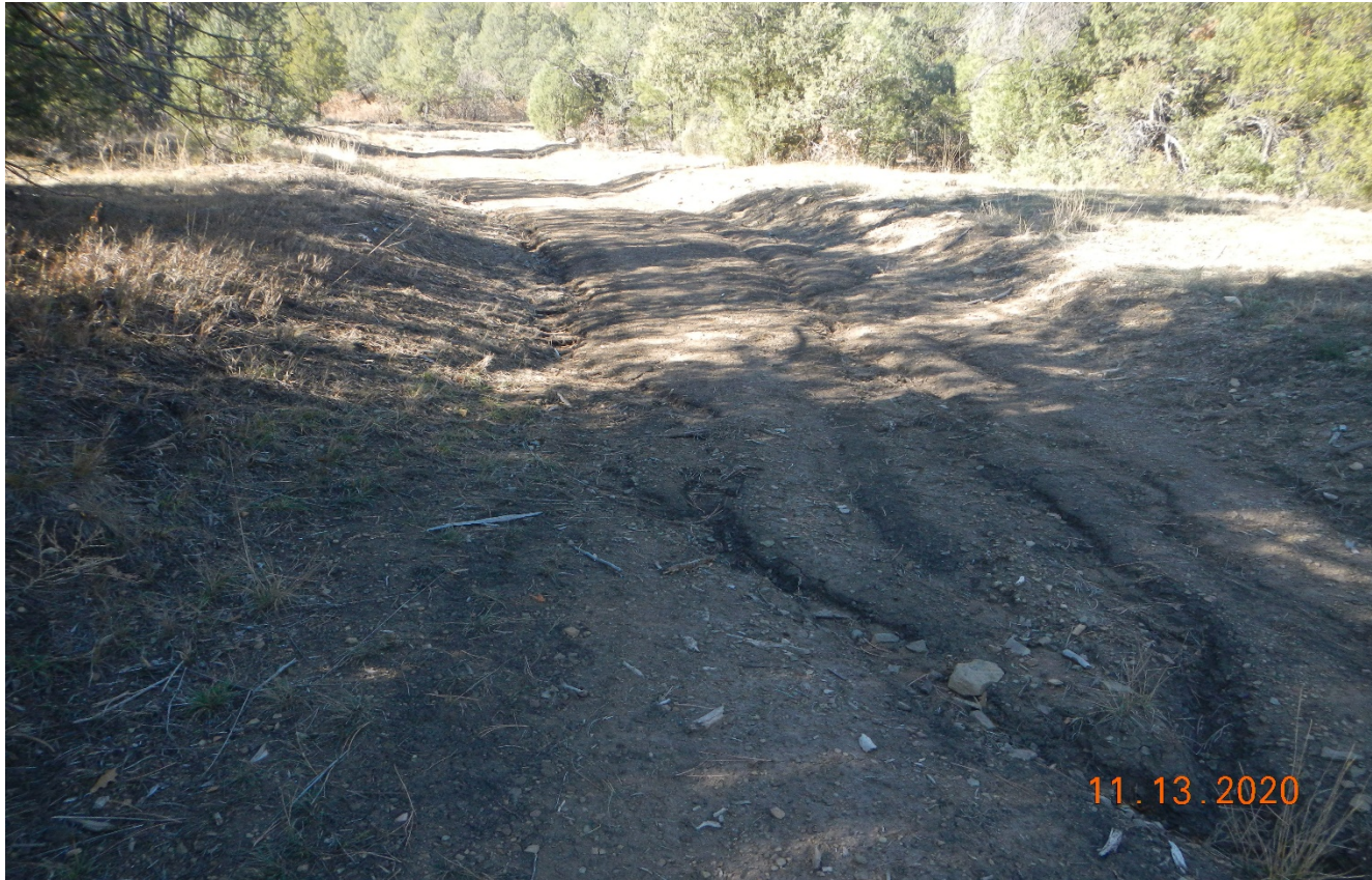
Photo 2. There is erosion rilling down the road that will need to be repaired.
