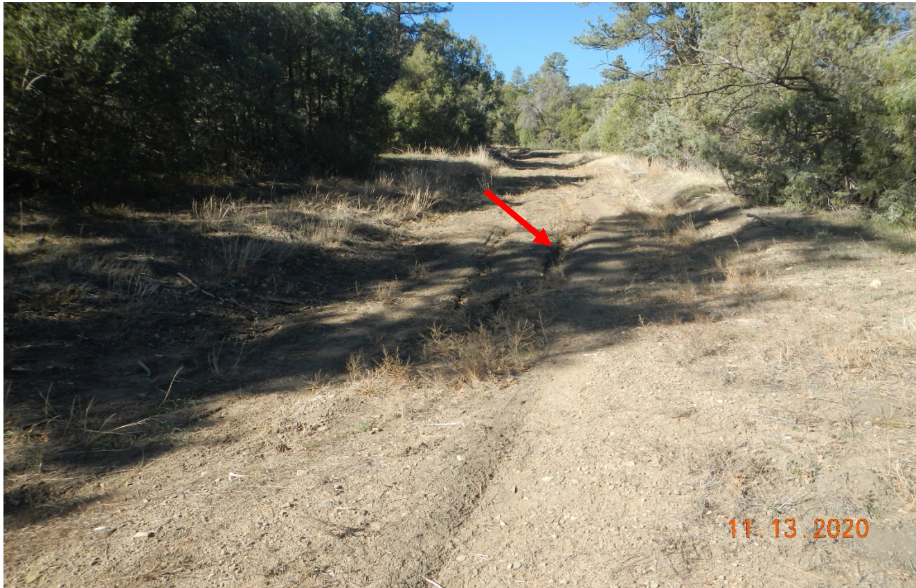
Photo 1. Facing northwest the beginning of the access road. The road appears to be pre-existing however, there are signs of stormwater erosion down the road.
