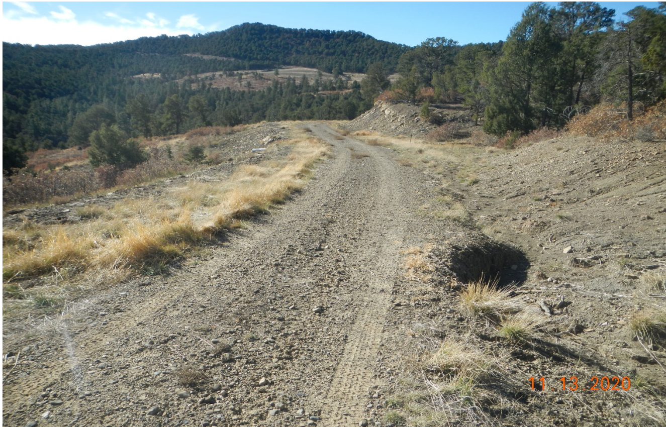
Photo 1. Facing southwest the beginning of the access road. The access road has not been recontoured and reclaimed.
