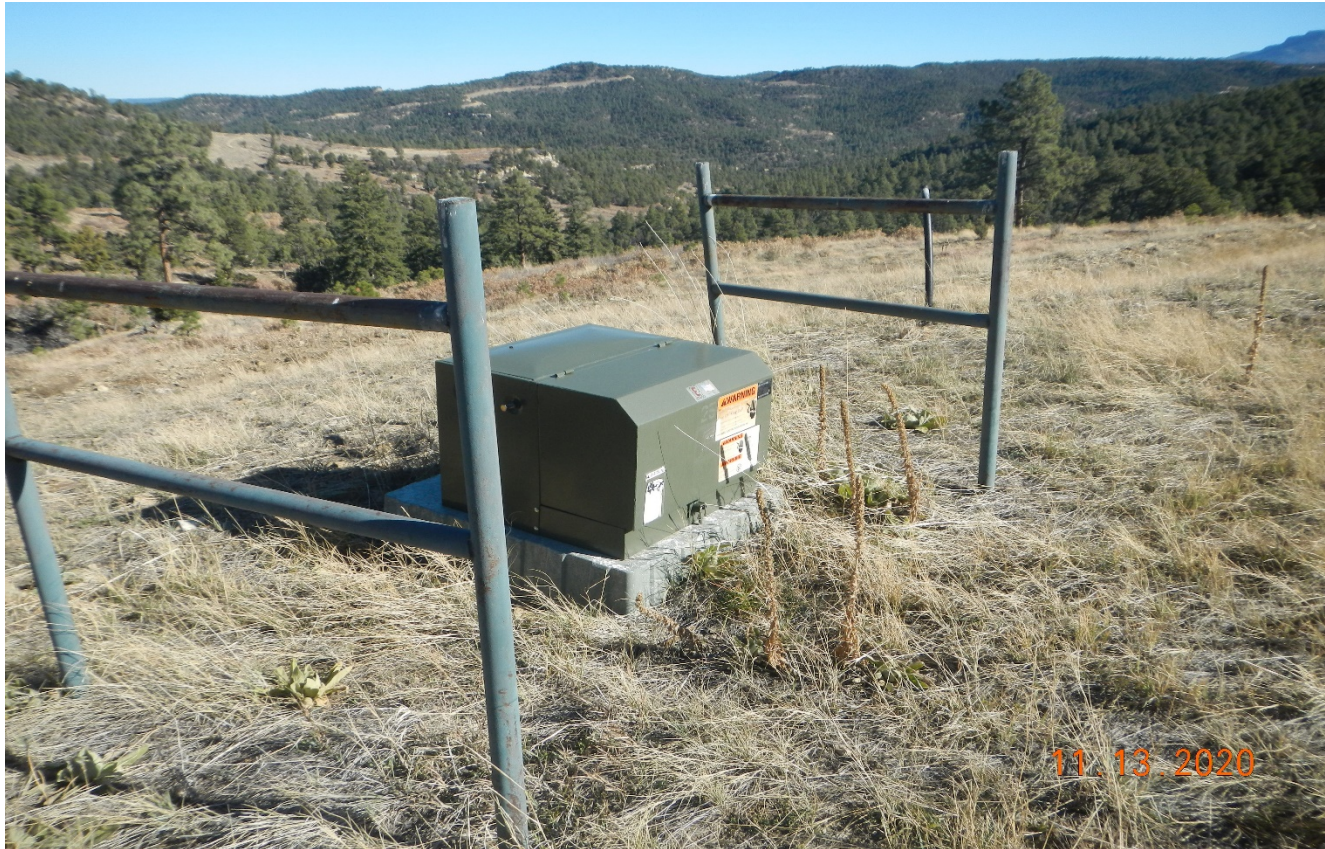
Photo 6. The electric utility has not been removed. There was a buzzing noise heard from the utility which indicates it active.
