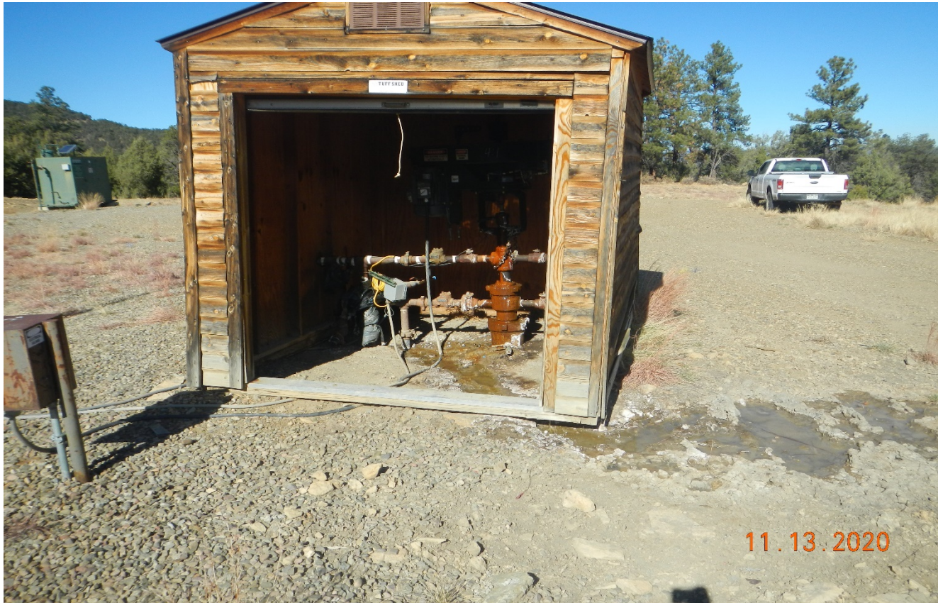
Photo 2. Facing inside well shed. There is a dripping water leak from the well head.
