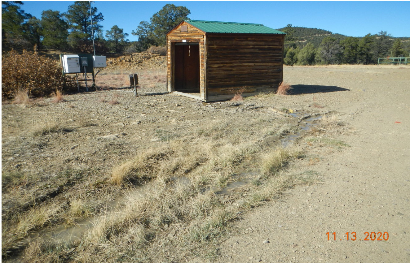
Photo 1. Facing toward the well which is inside the shed. There is water leaking from the well and flowing down the road.
