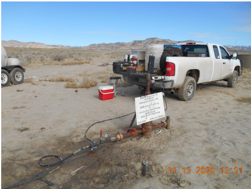
Wellhead during MIT operations
