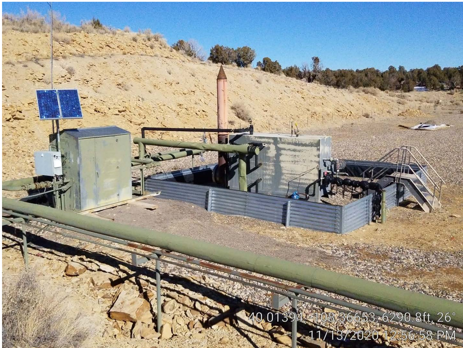
Photo 3. Meter building & separator.
