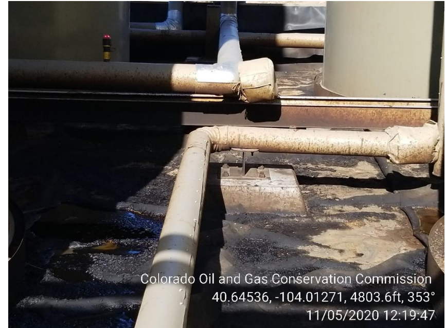
Photo 12 – Oily Waste at Produced Water Tanks
