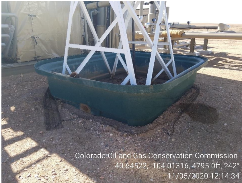
Photo 7 – Compressor Day Tank – Netting is in disrepair
