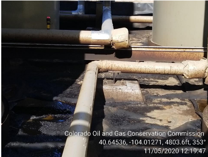
Photo 11 – Oily Waste at Produced Water Tanks
