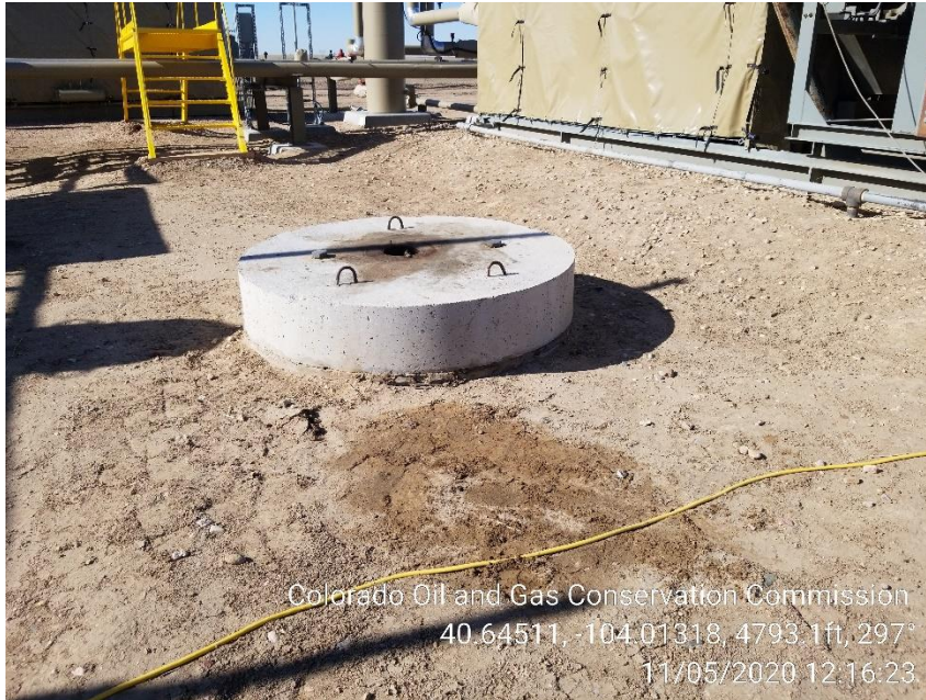
Photo 9 – Compressor Drain Pit – Missing Signage and Stained Soil
