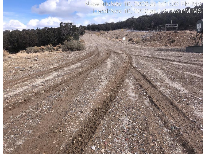
Photo #2234 Tracking occurring from location to access road.
