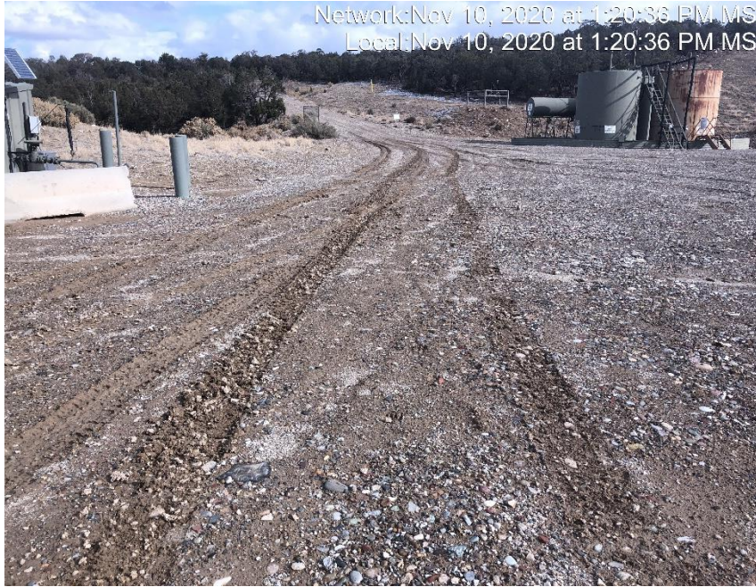
Photo #2233 Tracking occurring from location to access road.
