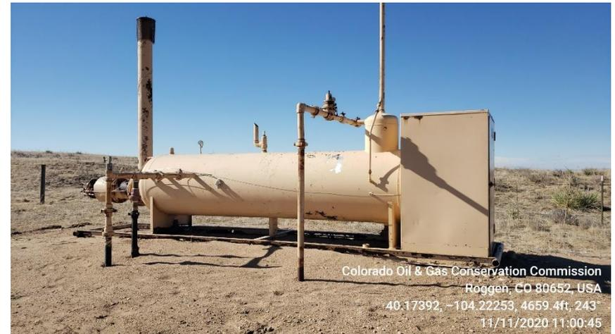
Photo 6 Horizontal Heated Separator.
