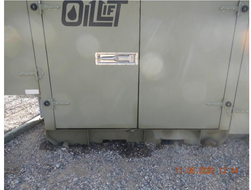
Stained gravel beneath Oil Lift equipment.
