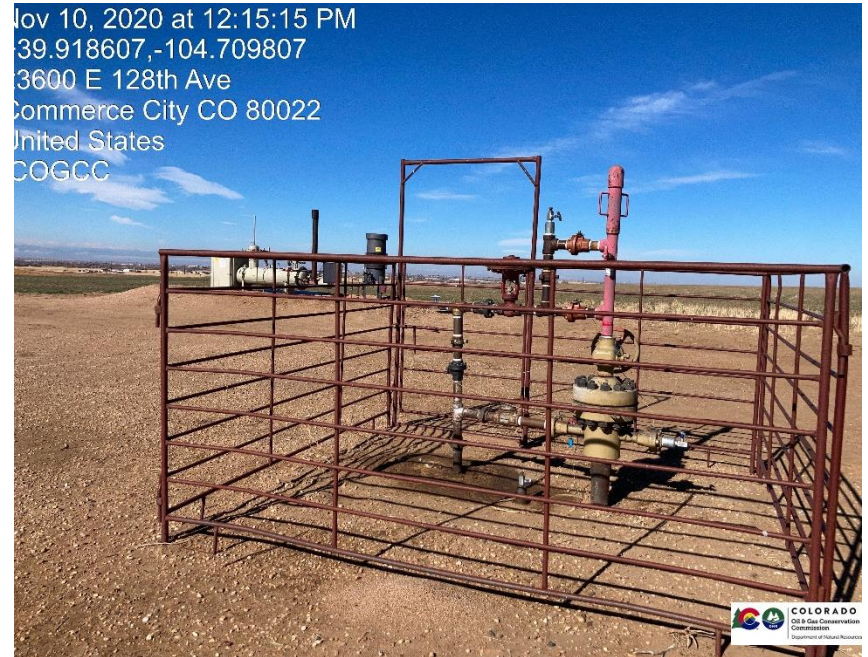
Pic 2 Stained soil / mechanical issues possible leak
