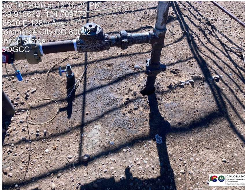
Pic 3 stained soil / mechanical / possible leak.
