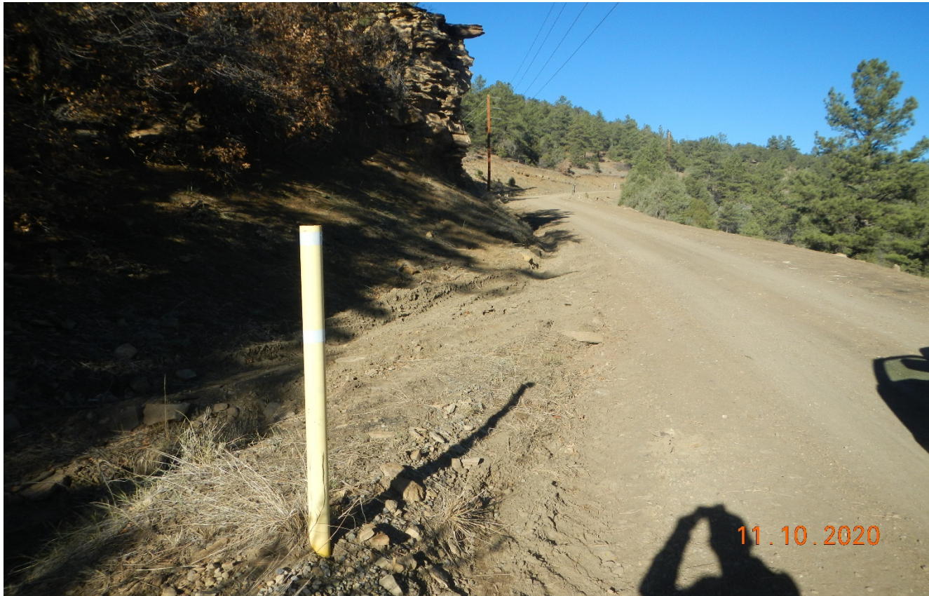
Photo 1. Facing southeast along the access road. The road has been regraded to divert stormwater toward the culvert.
