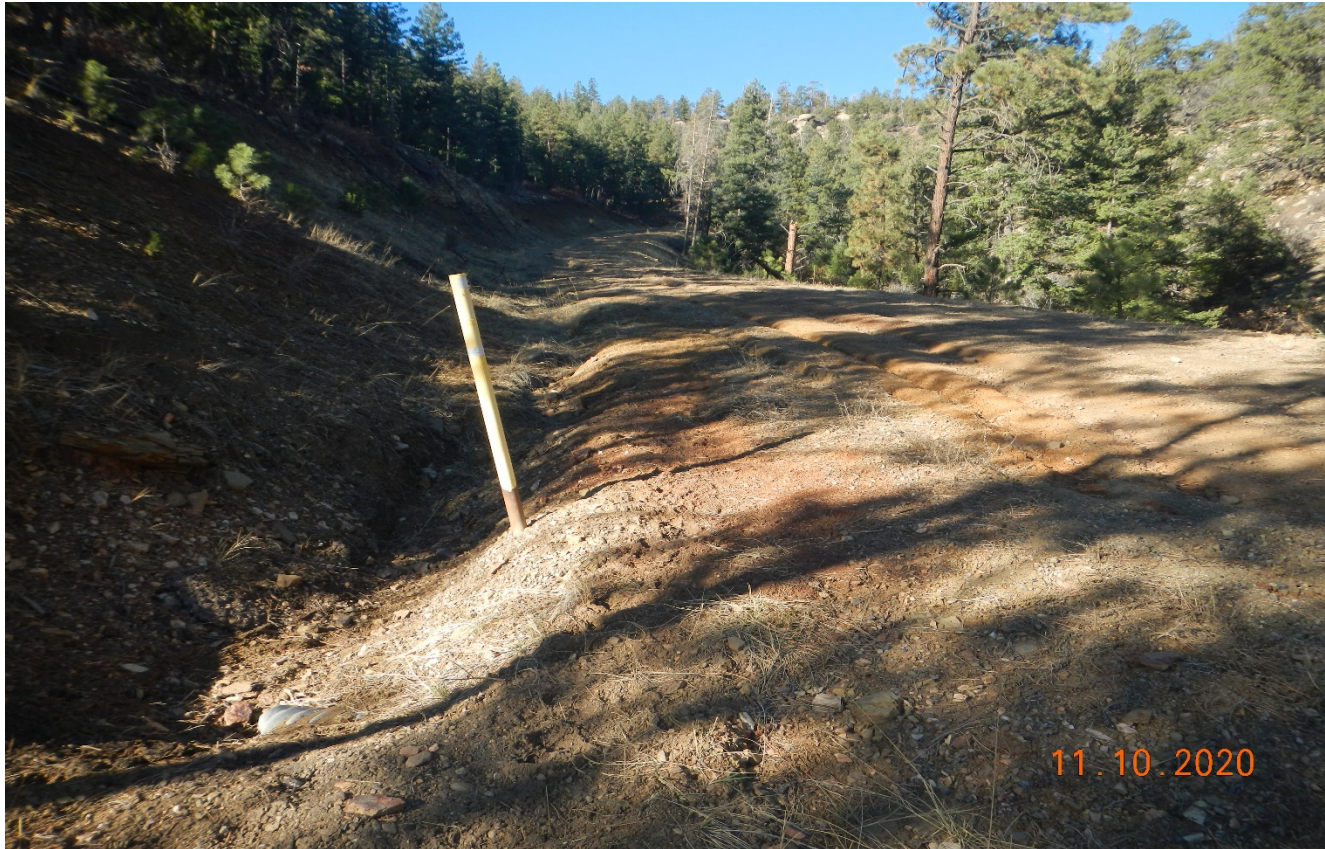
Photo 2. Facing northwest along the access road. There are culverts filled in with sediment and stormwater is not directed toward the culvert.
