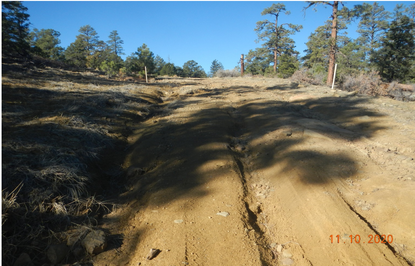
Photo 8. The road has eroded and needs to be repaired.
