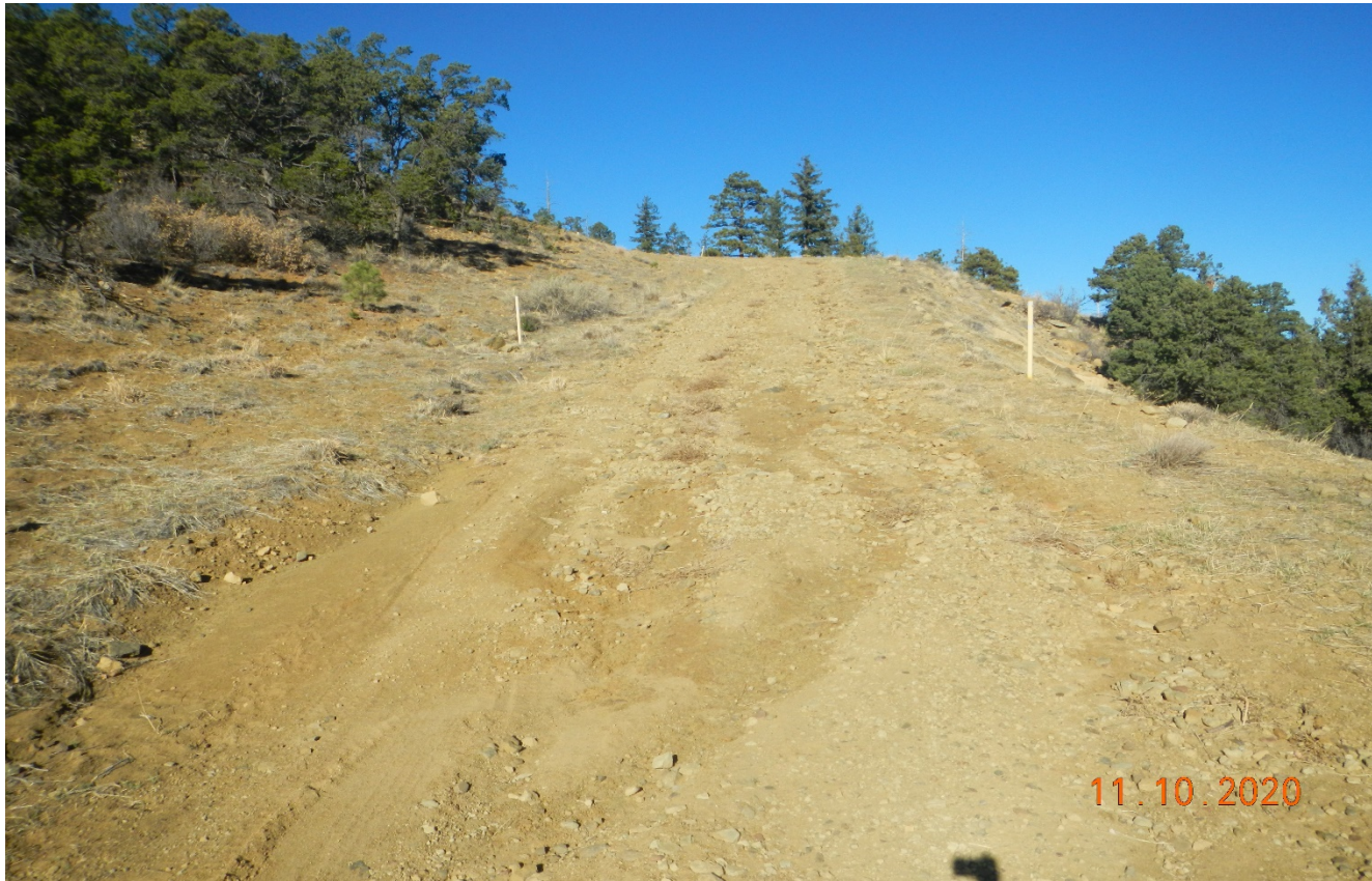
Photo 6. Facing northwest toward the location which continues past the location. There is erosion occurring down the road which is depositing sediment onto the location.
