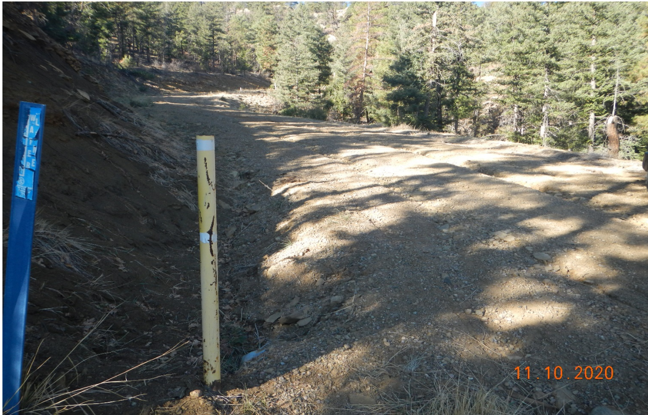
Photo 3. There are multiple culverts along the road filled in with sediment.
