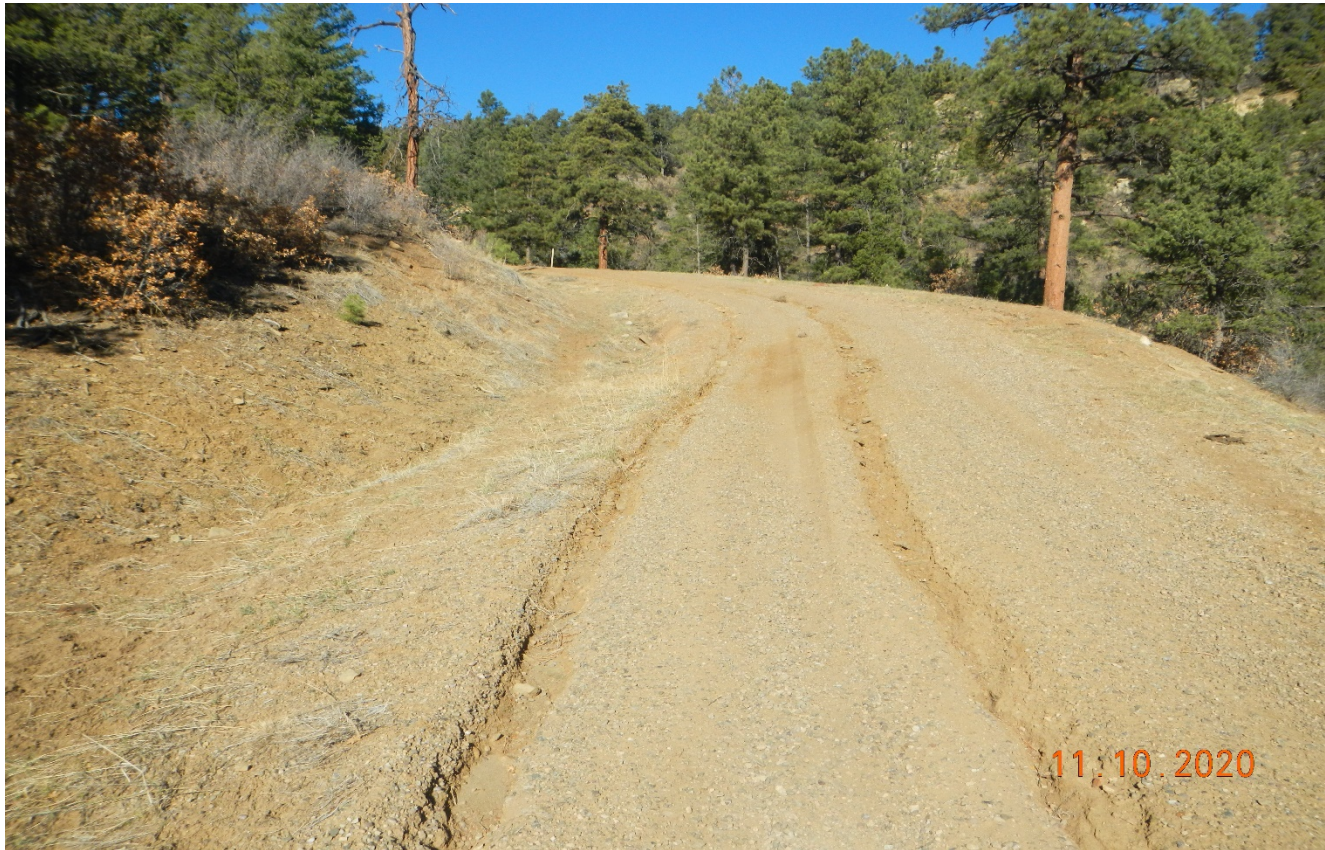
Photo 1. Facing northwest along the access road. There is erosion occurring down the road. Stormwater needs to be diverted toward the culverts.
