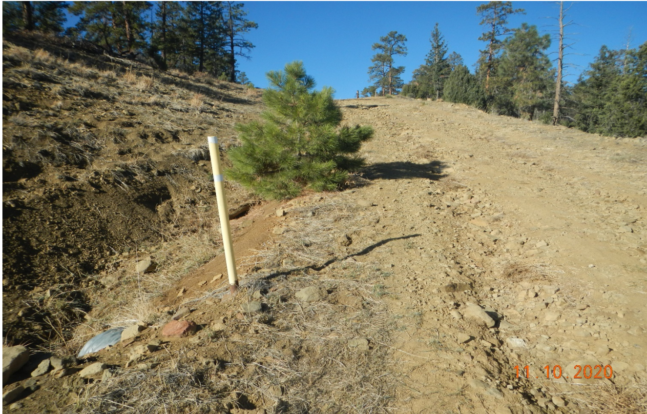
Photo 7. Stormwater is flowing down the road causing erosion and not diverted toward the culverts.
