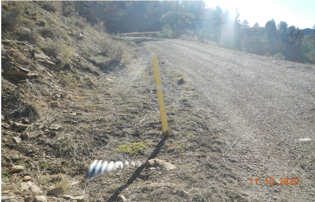
Photo 1. Facing southeast along the access road. There are multiple culverts along the road filled in with sediment.
