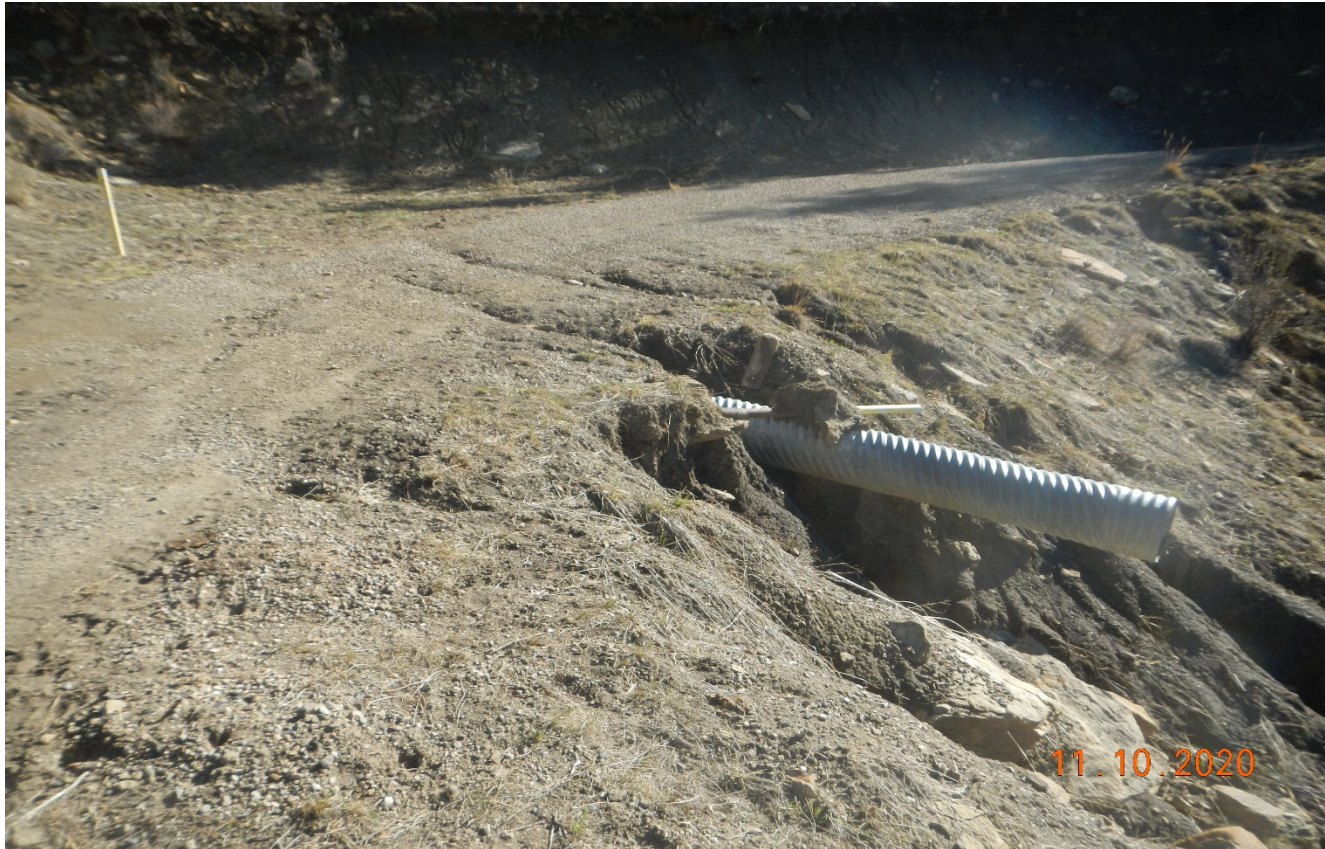
Photo 2. The culvert is filled in with sediment causing stormwater to flow across the road causing this erosion. The culvert stick out far creating a drop of stormwater and there is no outlet protection.
