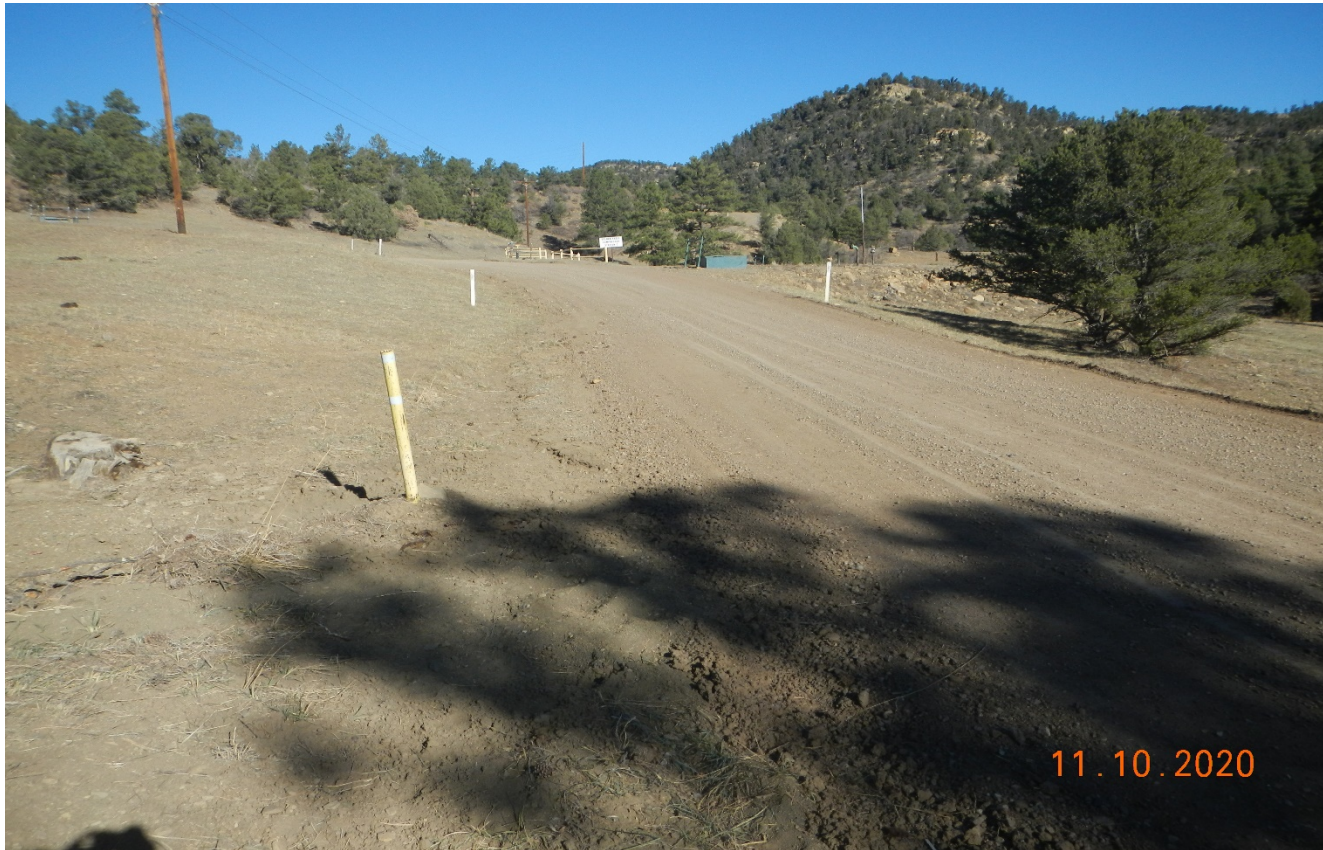
Photo 1. Facing northwest along the main access road. The culvert along the access road is filled in with sediment. Approx. Lat/Long:37.15036,-104.88730.
