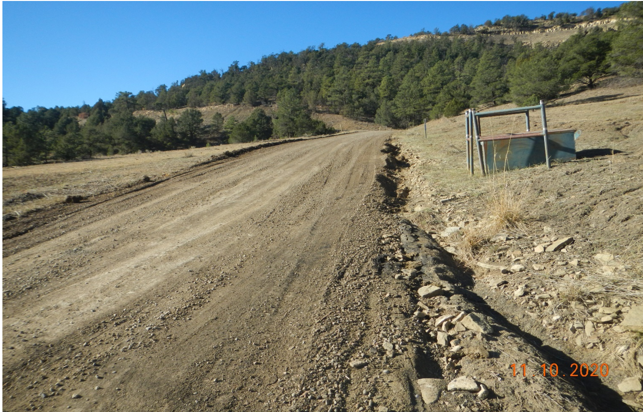
Photo 3. Facing southwest along the access road ascending the hillside. The road has been regraded. Additional BMP's are needed along the road side to prevent erosion.
