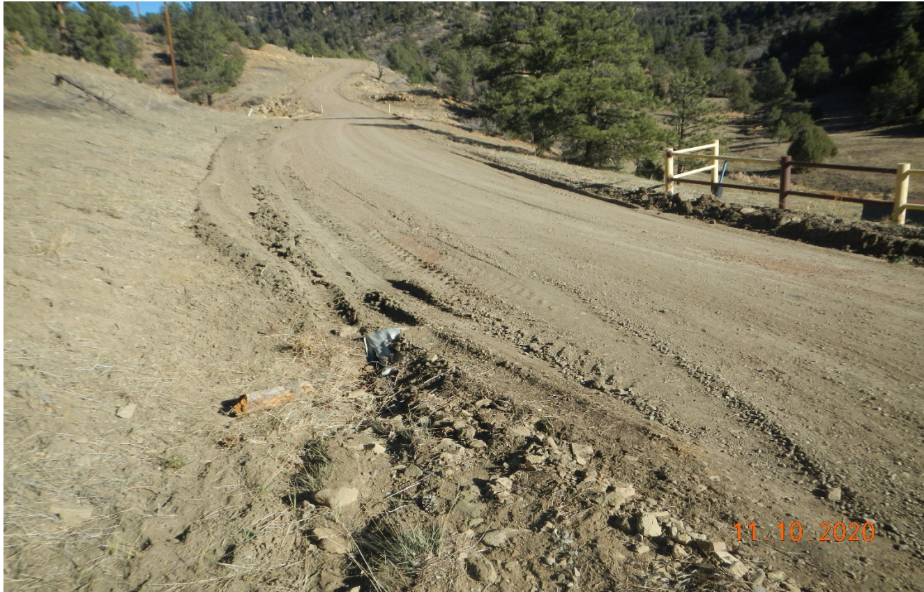
Photo 2. Facing north along the main access road. The culvert along the road is damaged. Lat/Long:37.15100,-104.88755.
