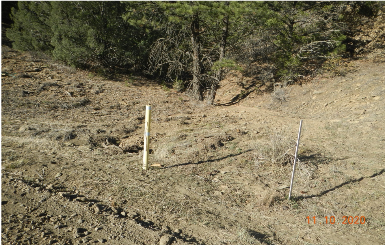
Photo 5. The culvert along the access road is filled in with sediment. Approx. Lat/Long:37.15042,-104.88852.
