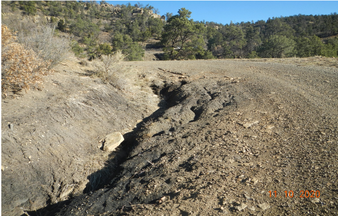
Photo 2. Facing northeast along the access road. There is erosion along the access road at Lar/Long: 37.15877,-104.88882. This area need to be repaired and stabilized.
