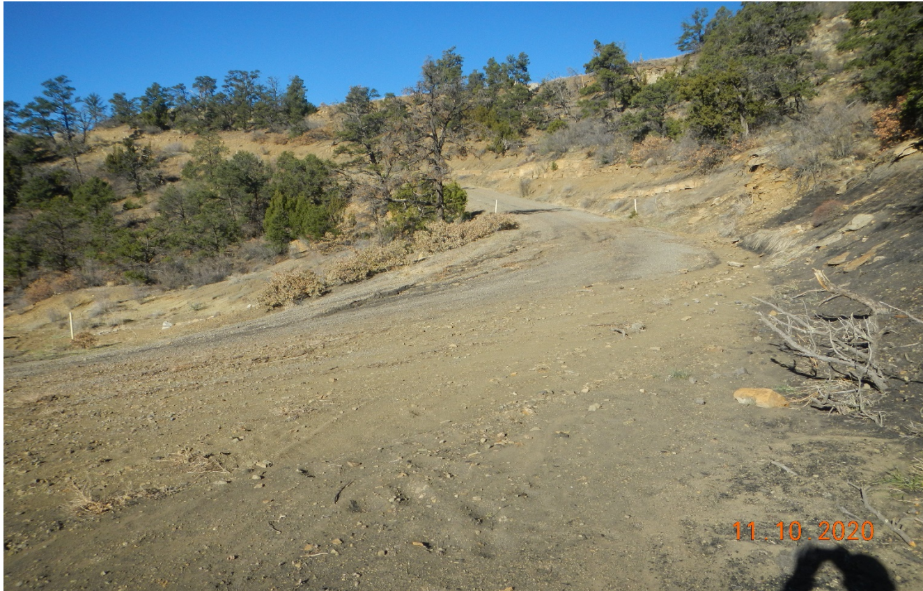
Photo 4. Facing northeast toward the access road. Stormwater is not flowing toward the culvert and is going across the road creating erosion shown in next photo. Previous corrective action has not been performed.
