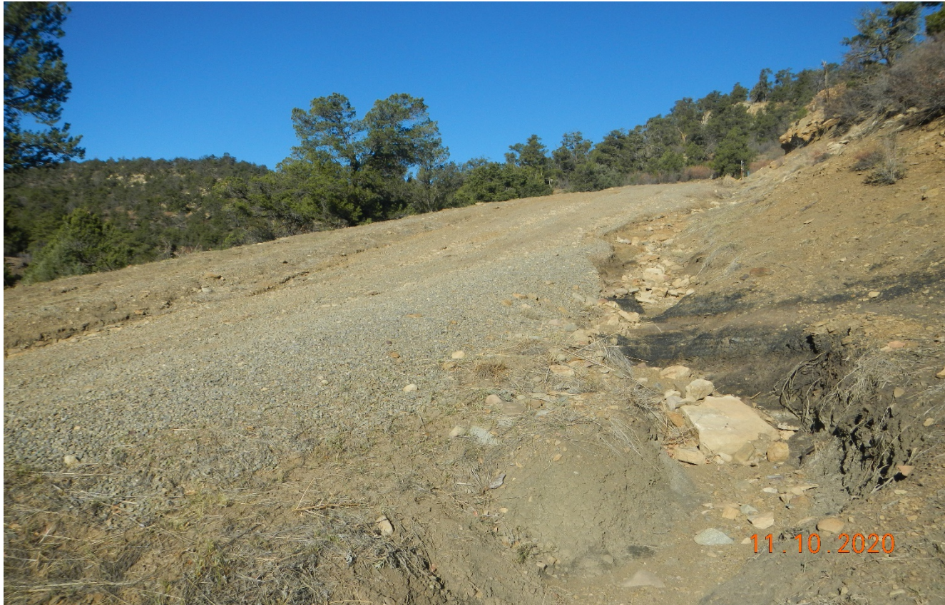
Photo 1. Facing northwest toward the access road. There is erosion along the access road at Lar/Long: 37.15772,-104.88855. This area need to be repaired and stabilized.
