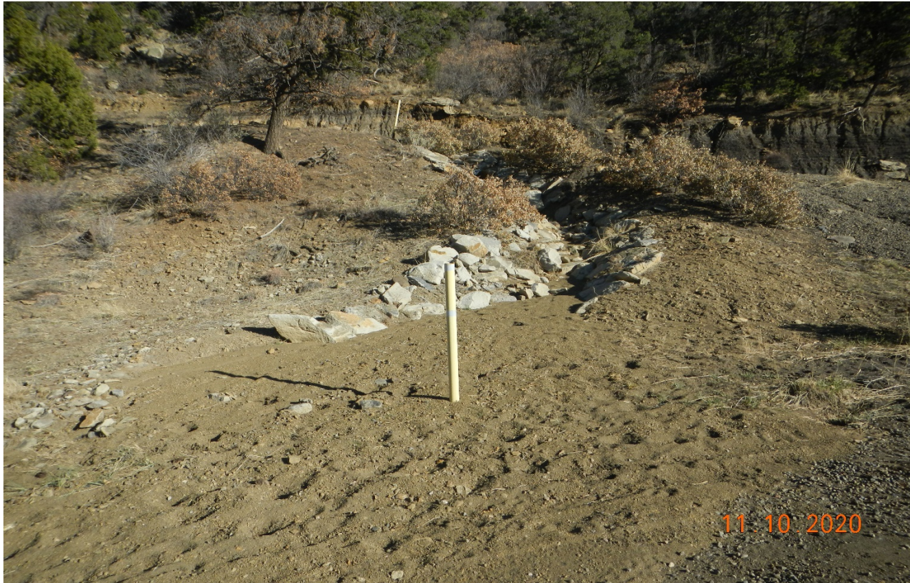
Photo 3. The culvert along the access road is filled in with sediment. Approx. Lat/Long:37.15953,-104.88851.
