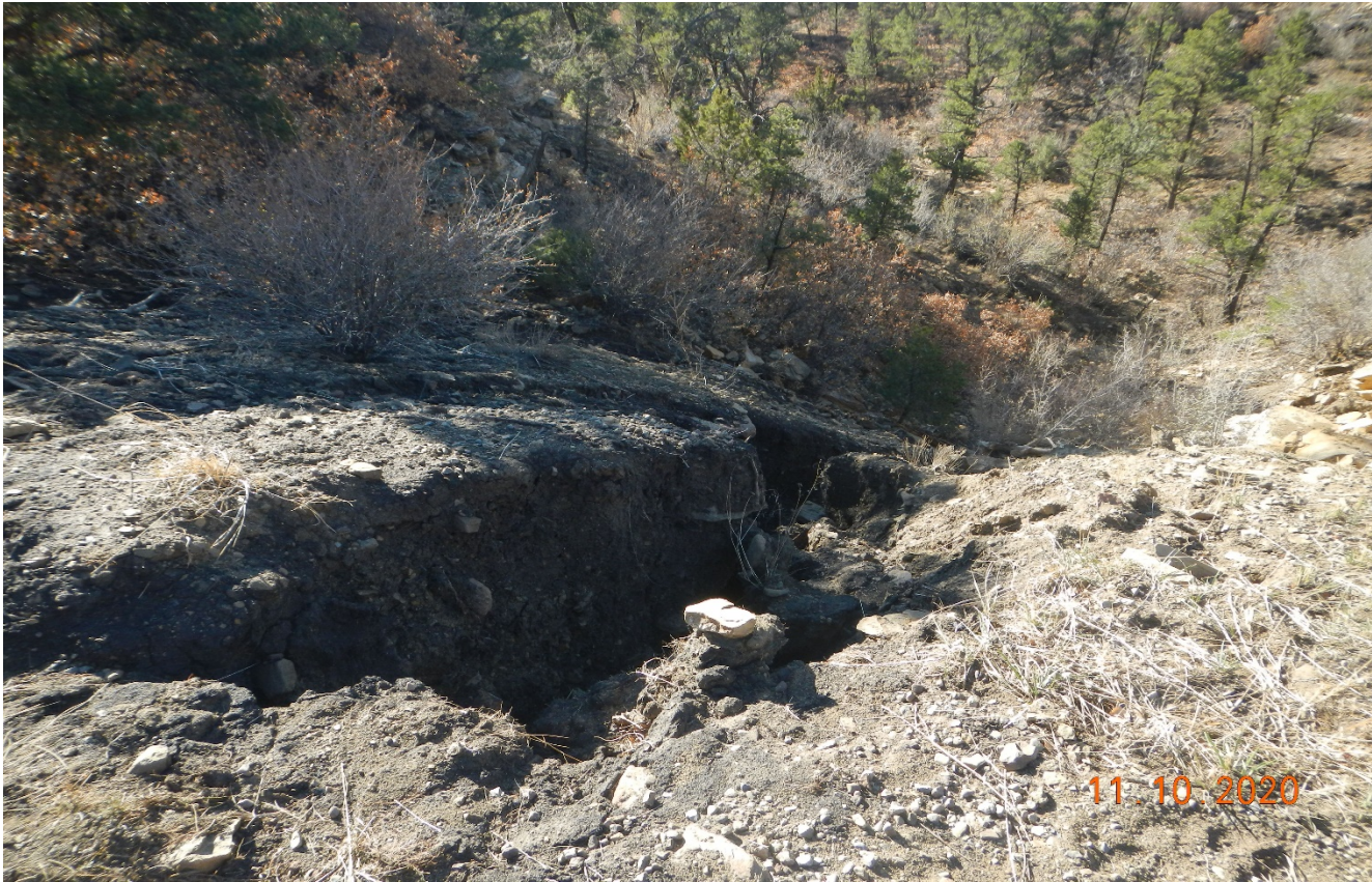
Photo 5. There is erosion occurring off the fill slope from stormwater flowing across the road shown in previous photo.
