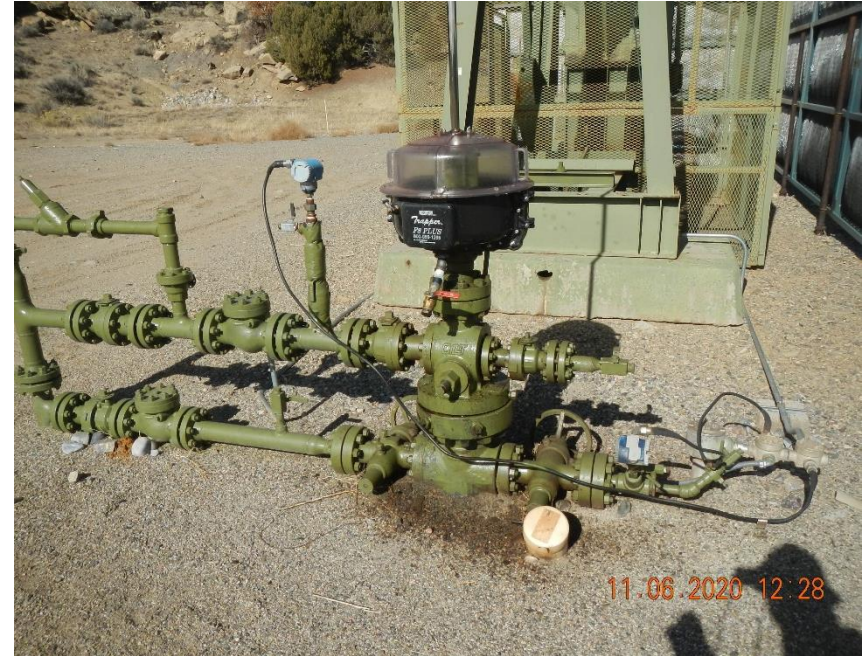
Well head is wet and surrounding gravel is wet and stained.
