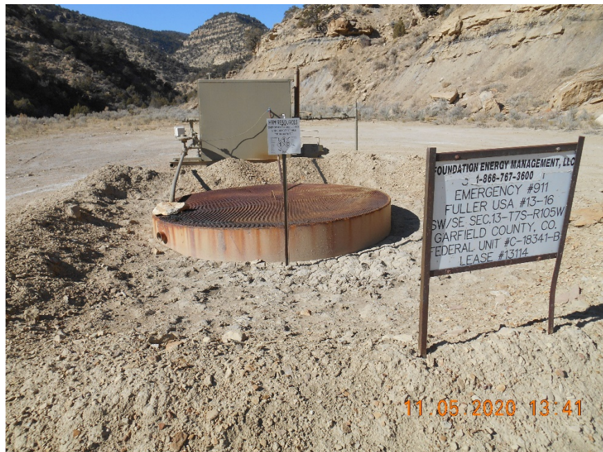
Separator and blowdown tank
