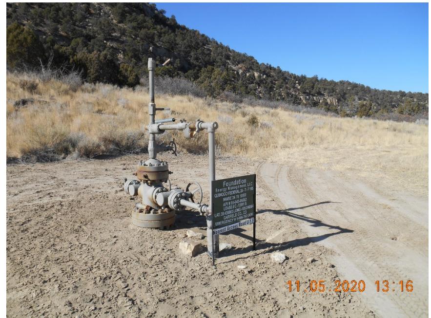
Wellhead with sign
