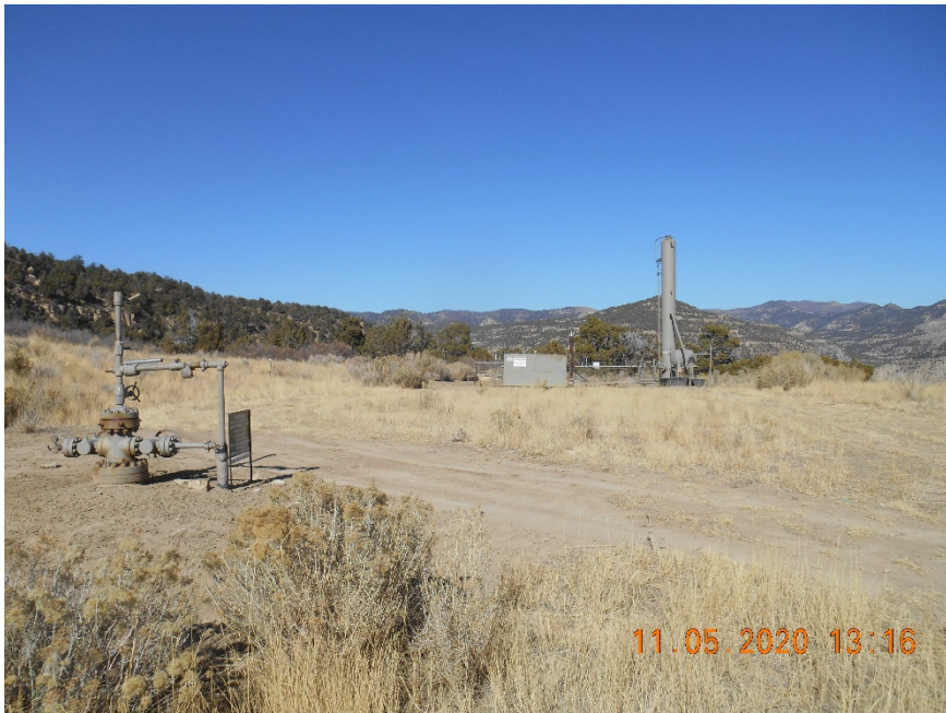
Location overview looking N.
