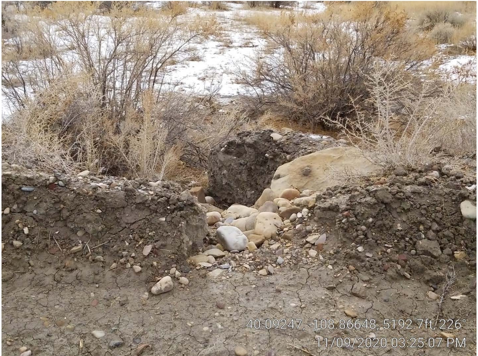
Photo 2. Stormwater channel through location edge berm.
