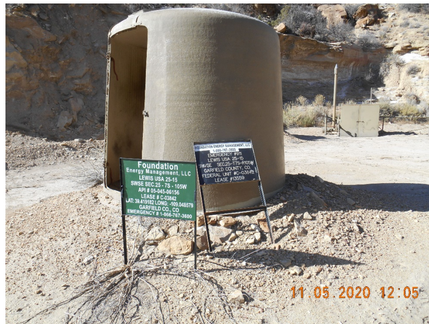
Wellhead inside housing with signs
