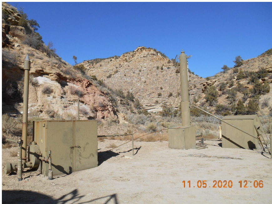
Separator, Dehydrator and Meter housing
