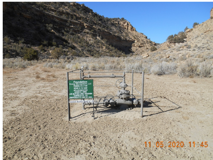
Wellhead with sign and fence
