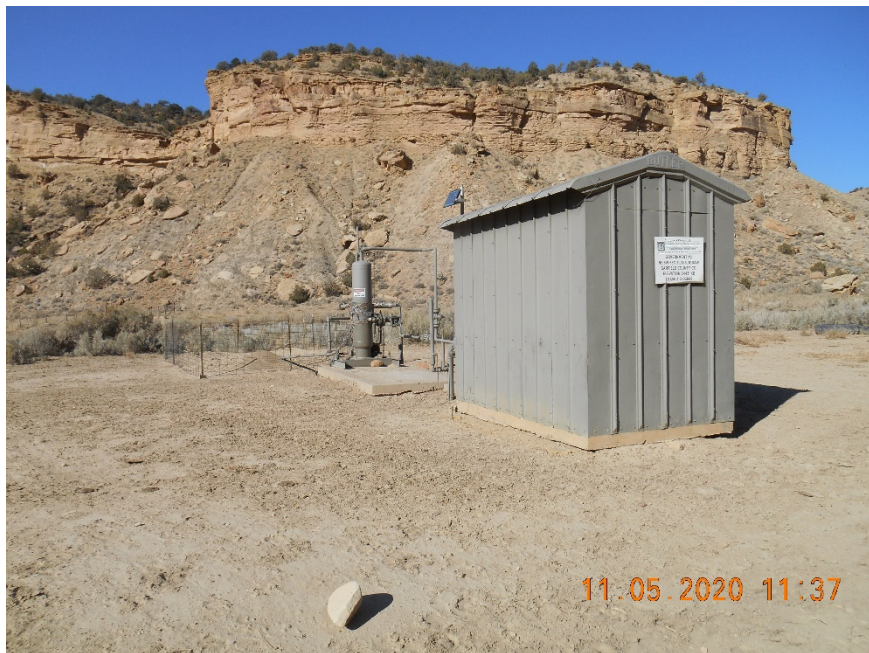
Meter housing and Separator
