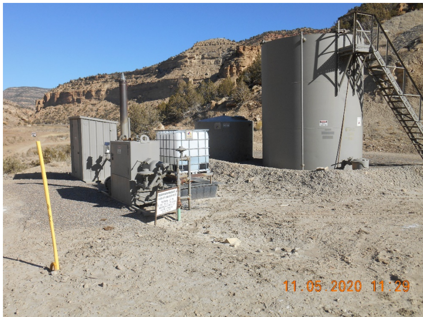
Separator, Meter housing and Tank Battery
