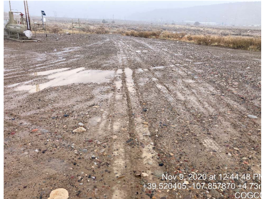
Lack of tracking controls
