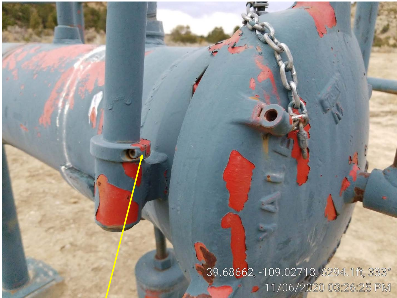
Photo 4. Gas leak at pig station.
