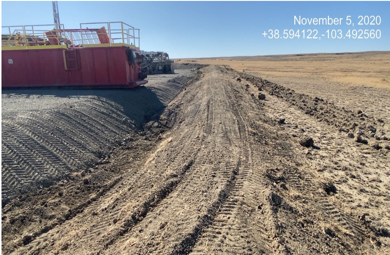
Photo 8. Facing northeast at the west side of the location.
