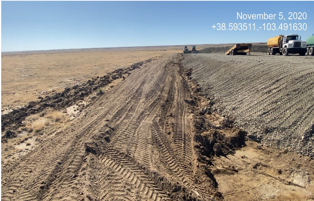
Photo 5. Facing southwest on top of the topsoil berm.
