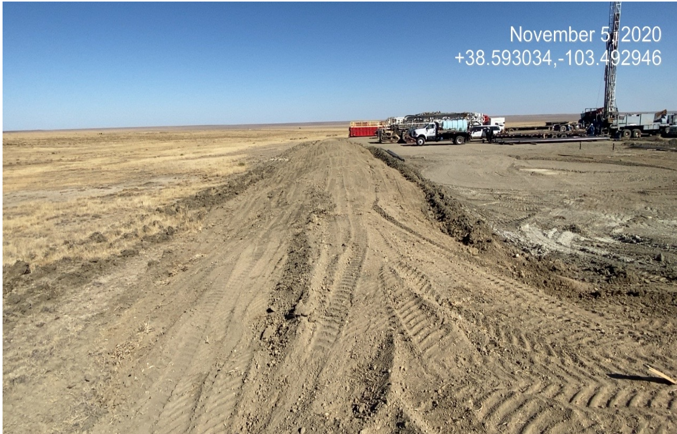
Photo 7. Facing northeast at the west side of the location.
