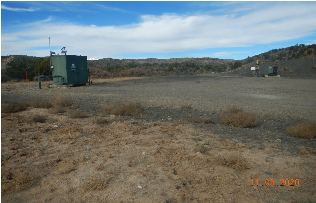
Photo 1. Facing northwest at the location.
