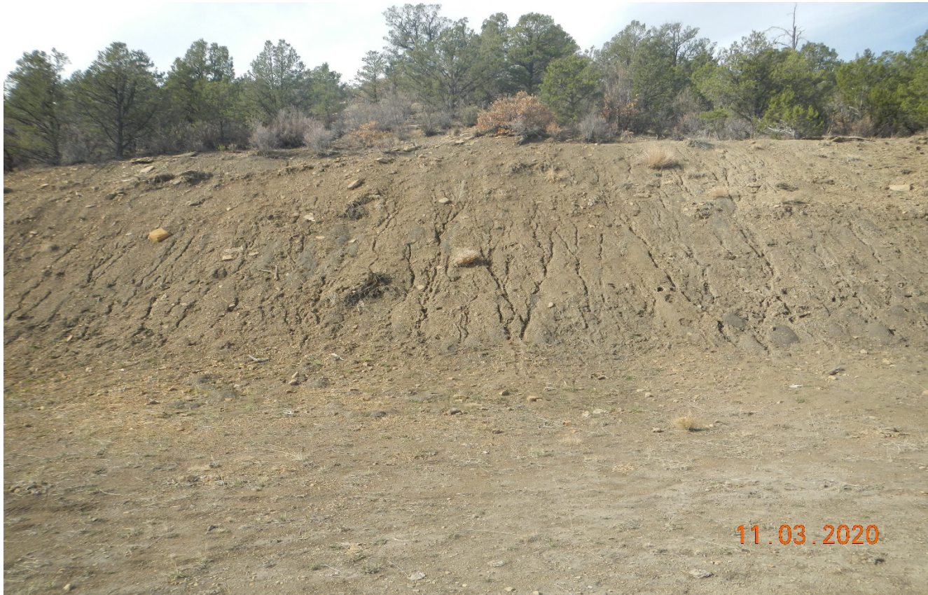
Photo 10. There is signs of erosion occurring off the cut slope.
