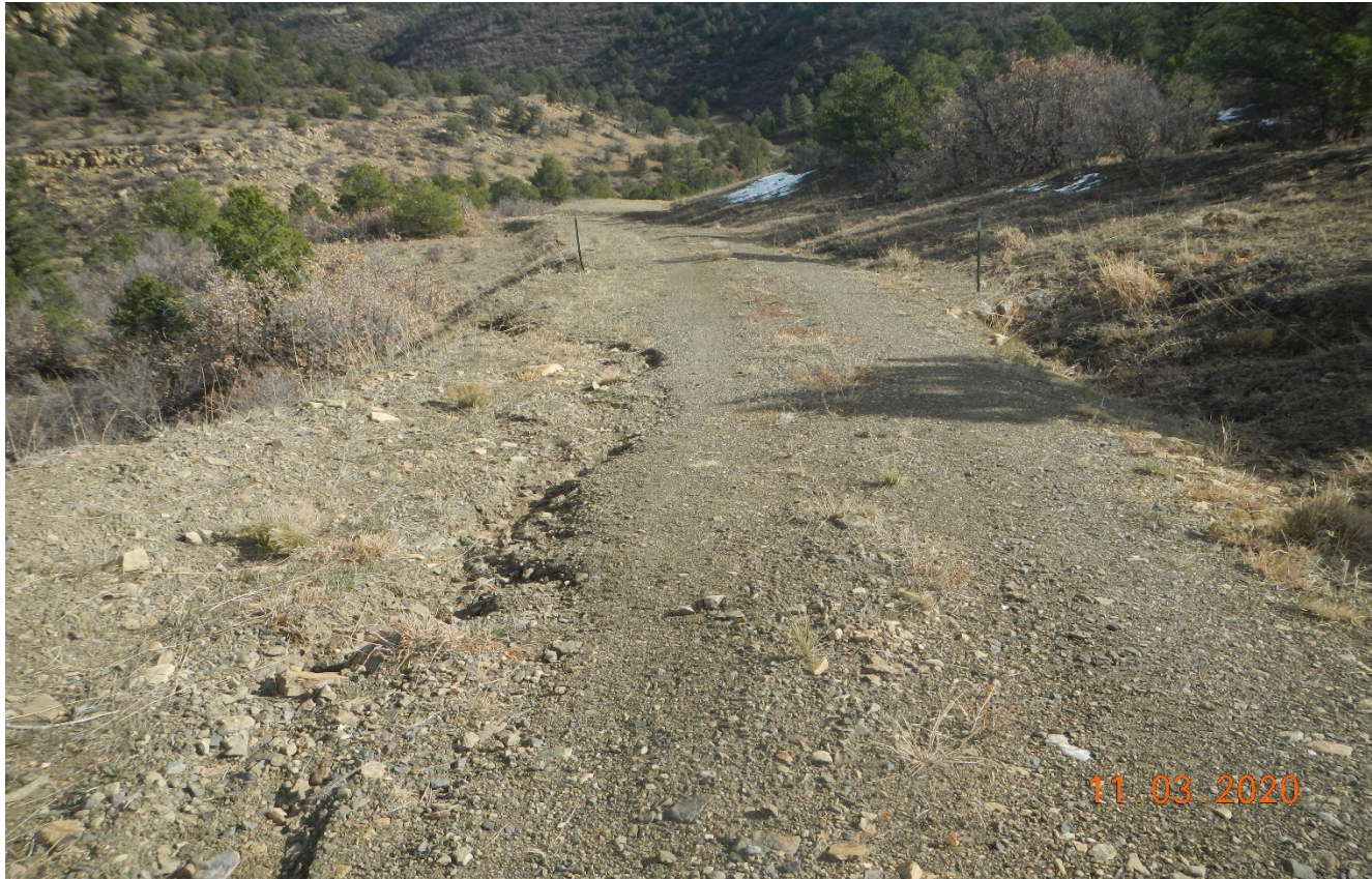
Photo 3. Facing east along the access road. There is an erosion channel along this area.
