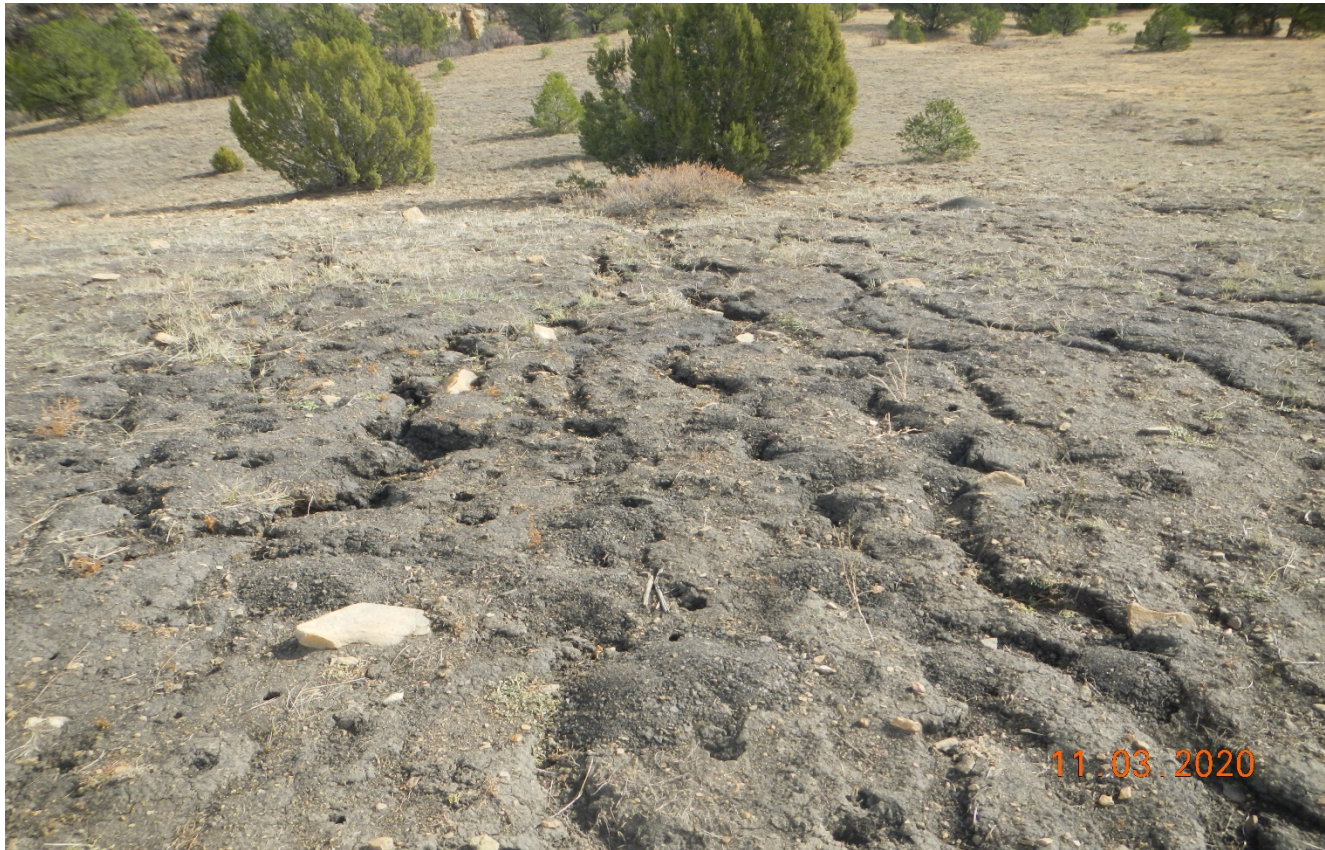
Photo 8. There is signs of erosion occurring off the fill slope.
