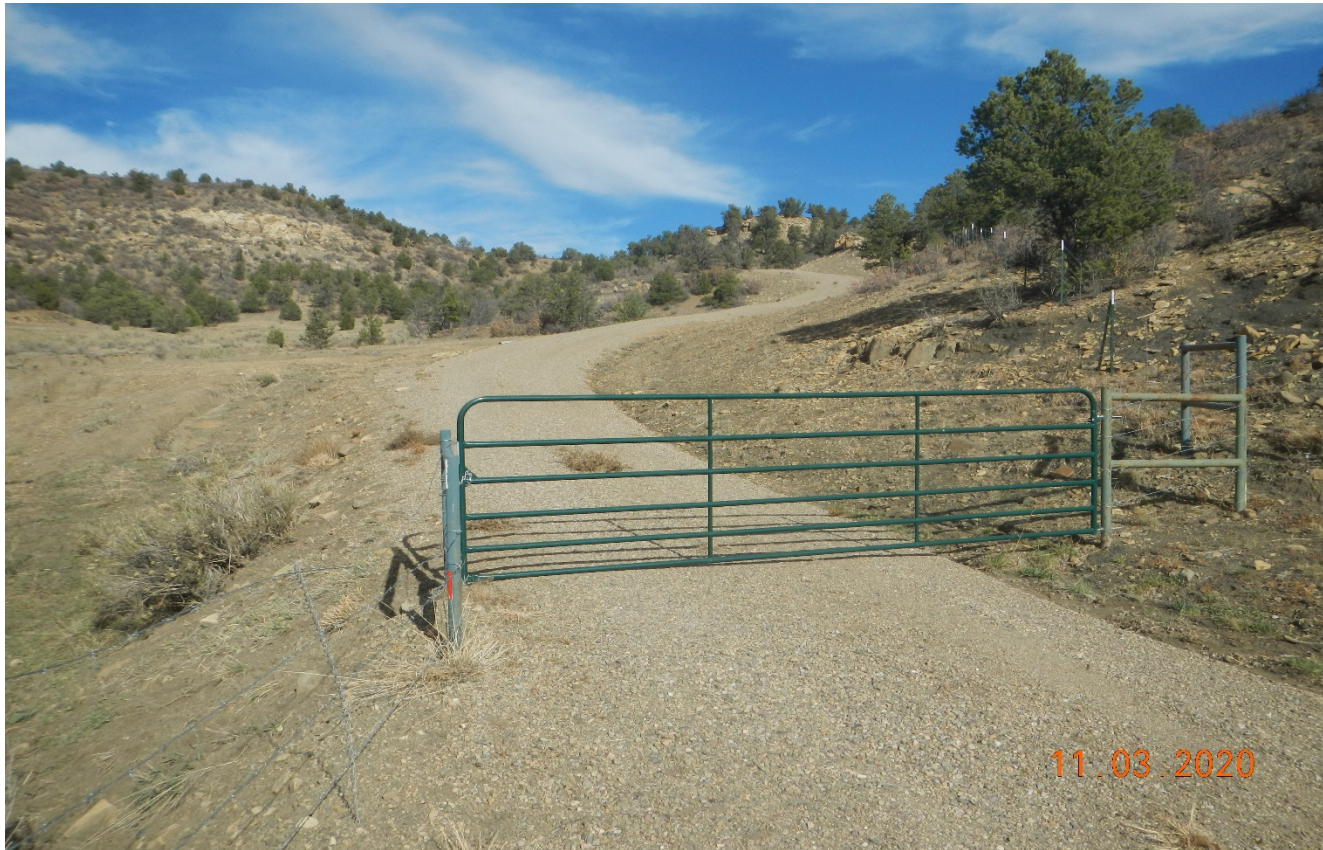
Photo 1. Facing north at the beginning of the access road. The road has not been recontoured and reclaimed.
