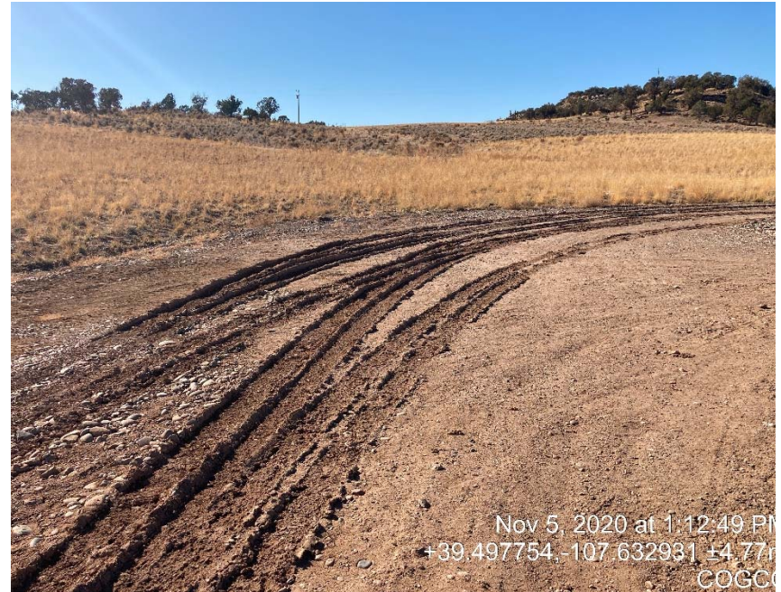
Rutting which will lead to tracking
