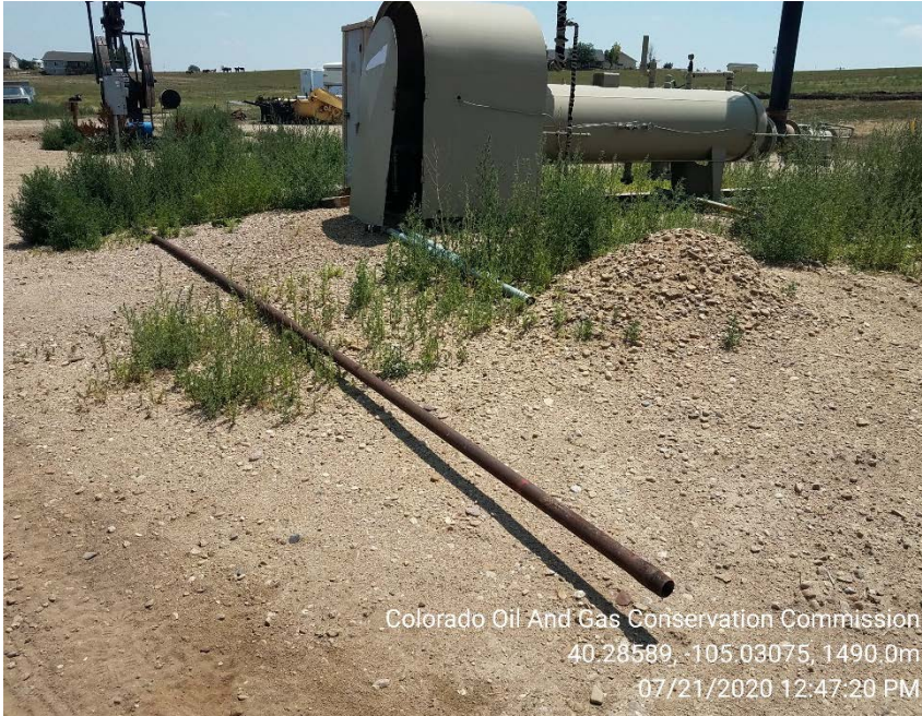
Unused equipment on 7/21/2020
