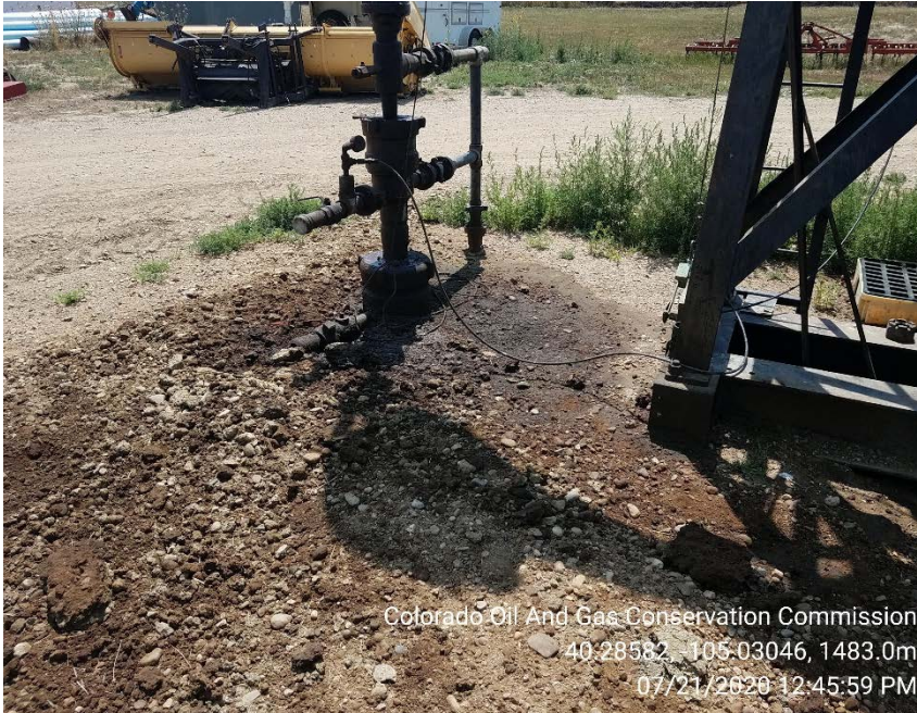
Stained soil on 7/21/2020
