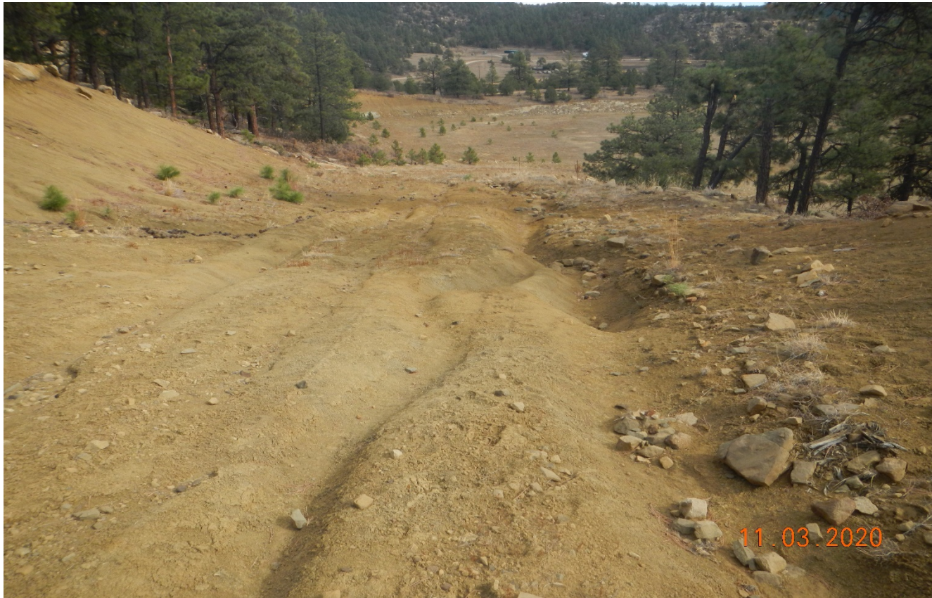
Photo 2. Facing east along the access road. There is erosion occurring down the road which is not stabilized.
