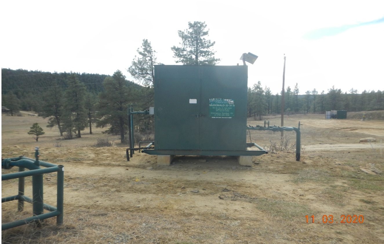
Photo 2. Well sign posted at meter shed.
