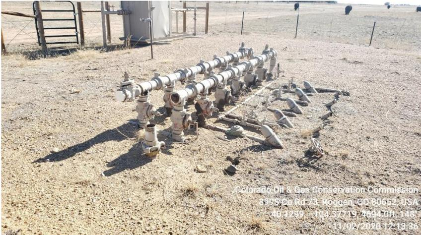
**Photo 9 Flow line manifold**
