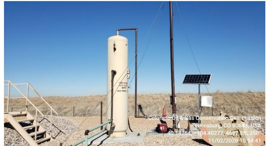
**Photo 5 gas meter run vertical heated separator**
