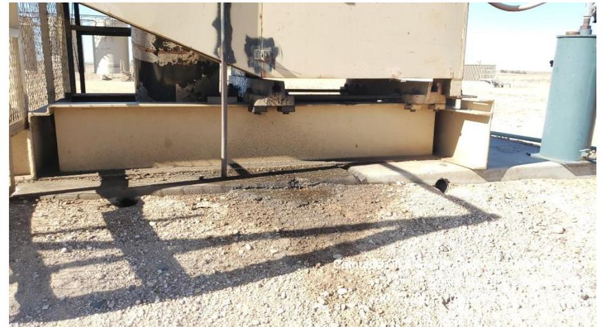
**Photo 3 stained soil by gas engine**
