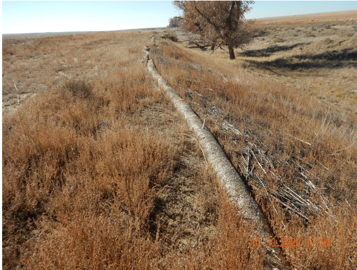
Photo 2. Photo taken from the associated offsite tank battery, facing South. Photo illustrates straw wattle BMPs installed in response to a previous corrective action inspection. Vegetation shown is Kochia and Russian thistle.
