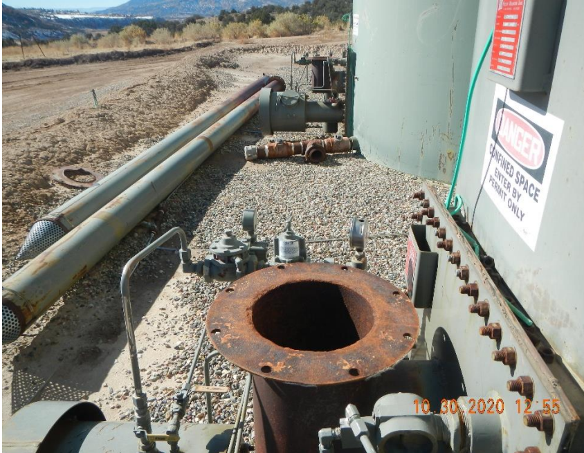
2 out of service 500 bbl heated tanks with stacks off of the heat units.
