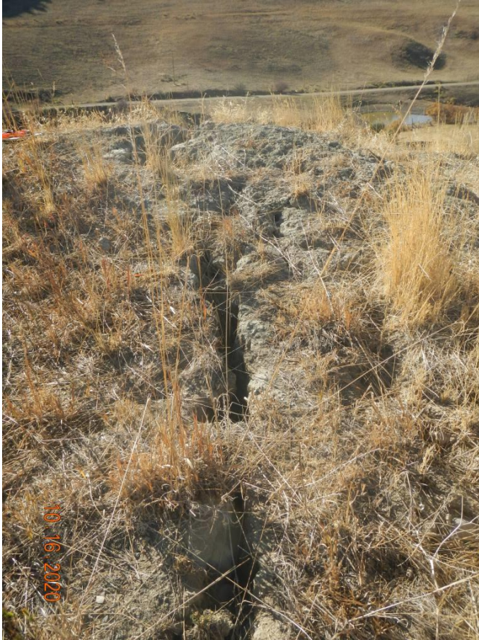
Photo#10: Erosion developed at NW corner of Fill.
