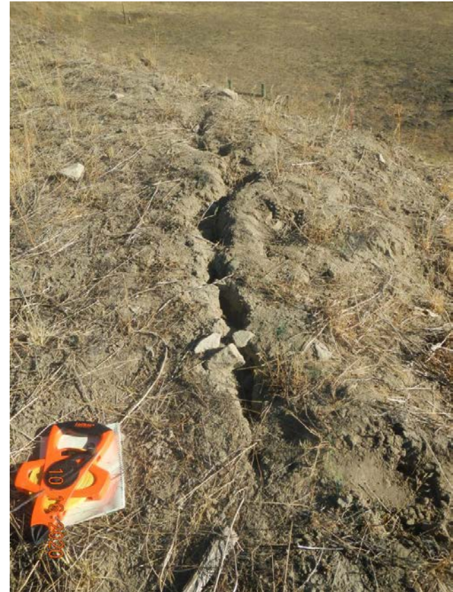
Photo#9: Cracking at top of fill at West side.
