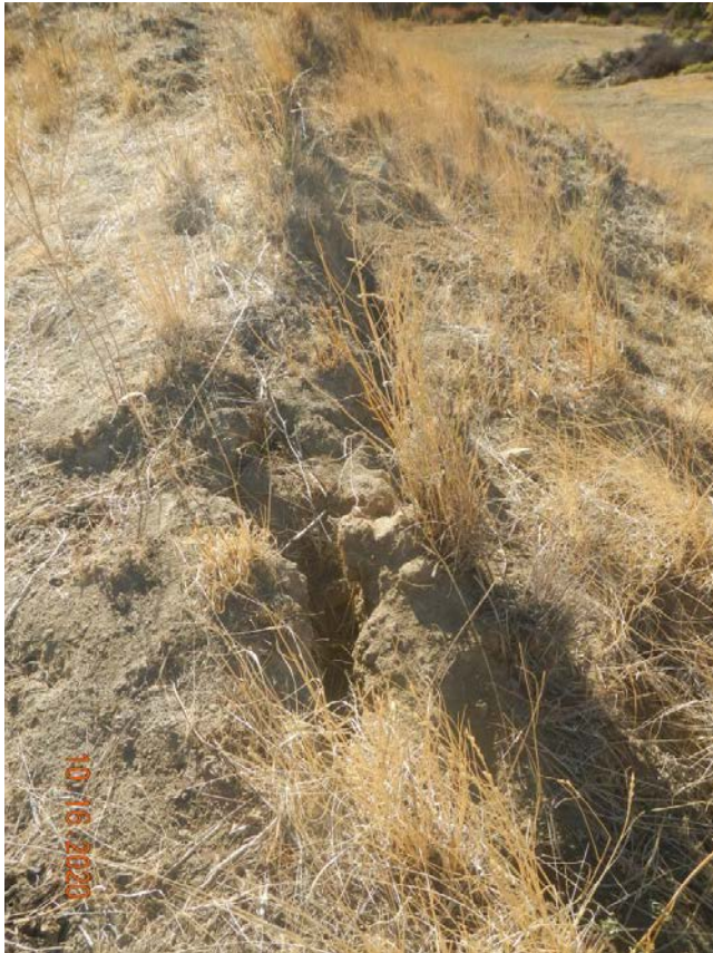
Photo#8: Cracking at top of fill at Northwest side.
