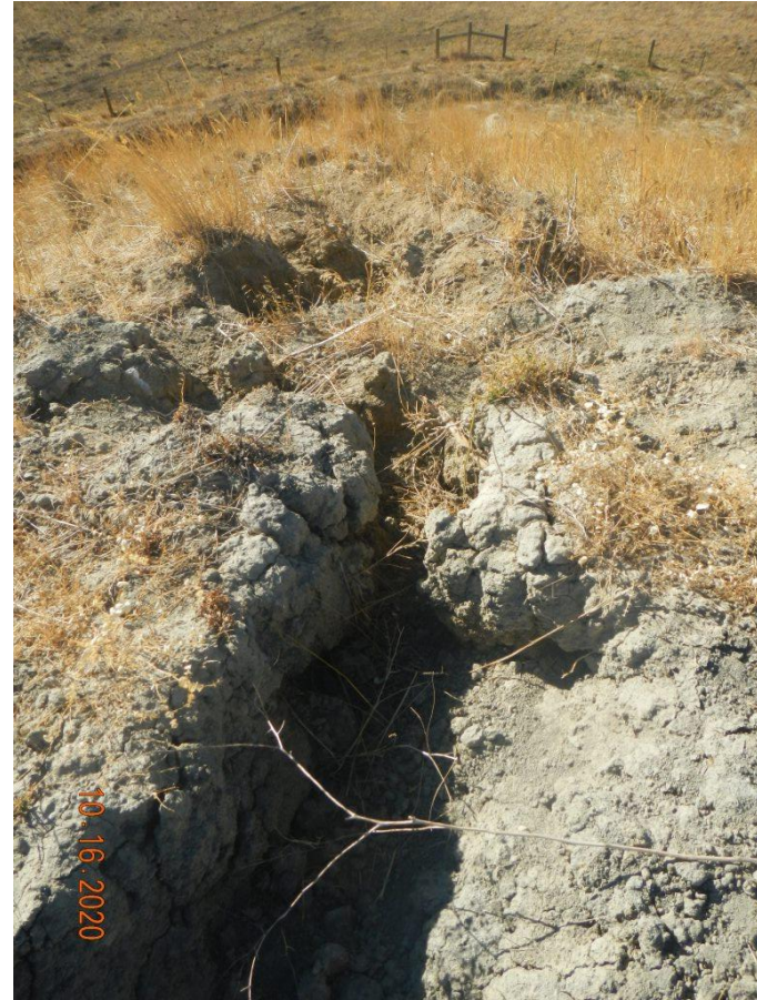
Photo#11: Erosion developed at NW corner of Fill.
