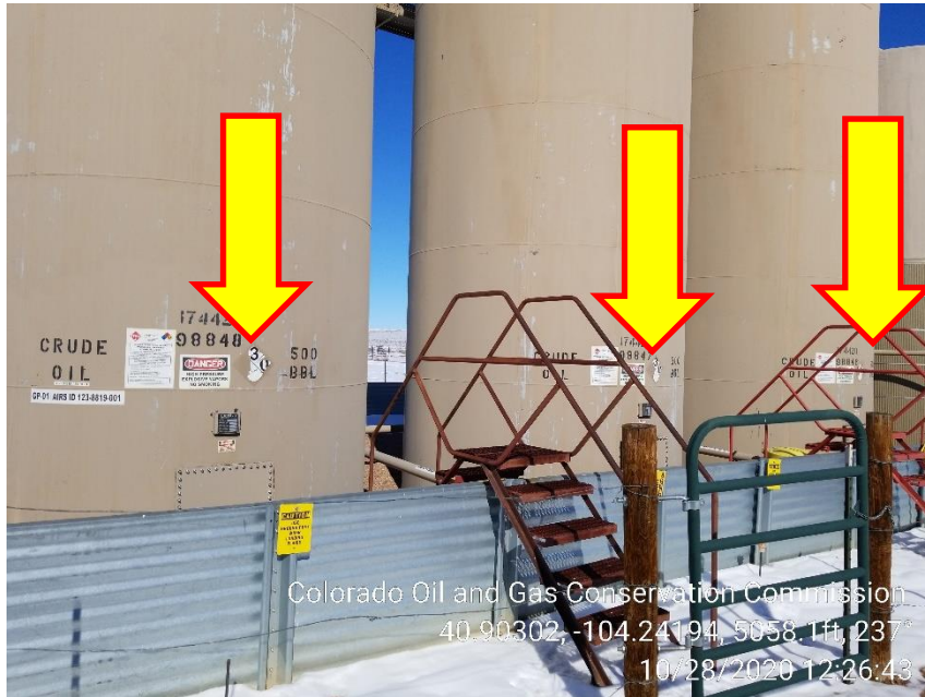
Photo 3 – Crude Oil Tanks missing NFPA Labels
