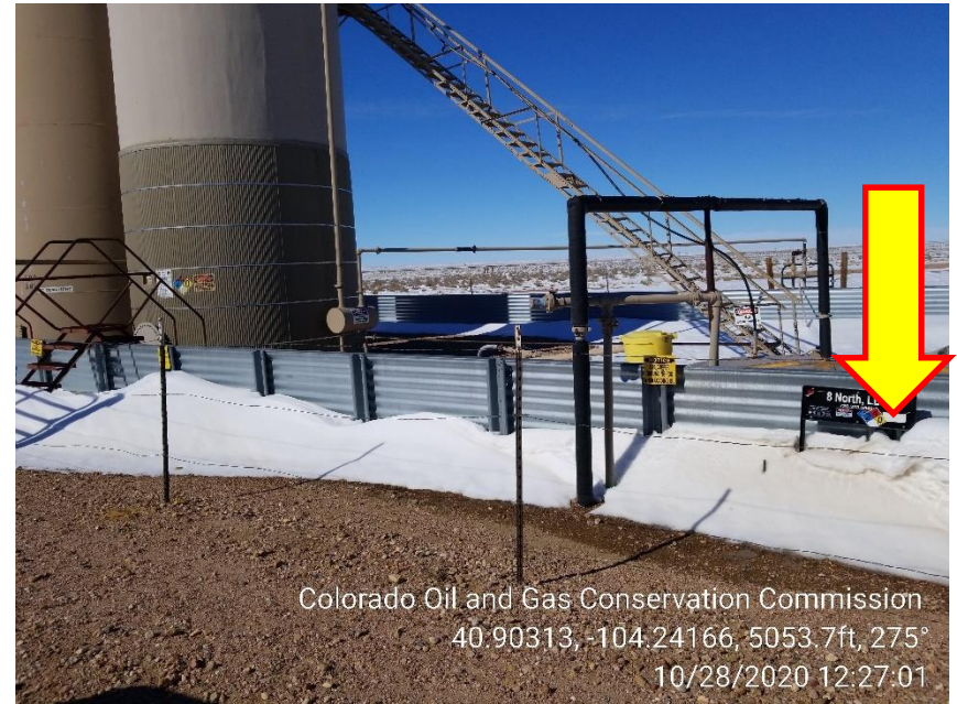
Photo 4 – Produced Water Tank missing Capacity Label
