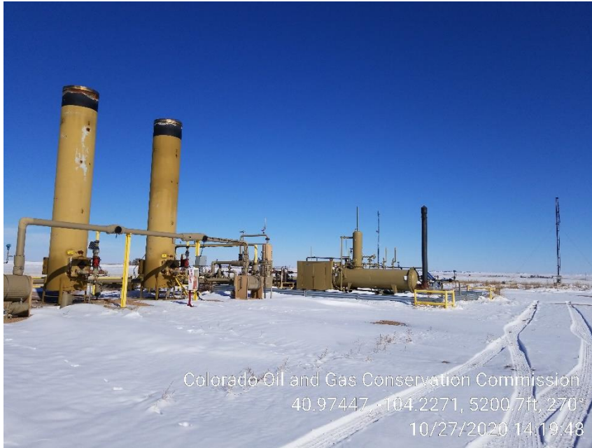
Photo 7 – Separator, ECDs
