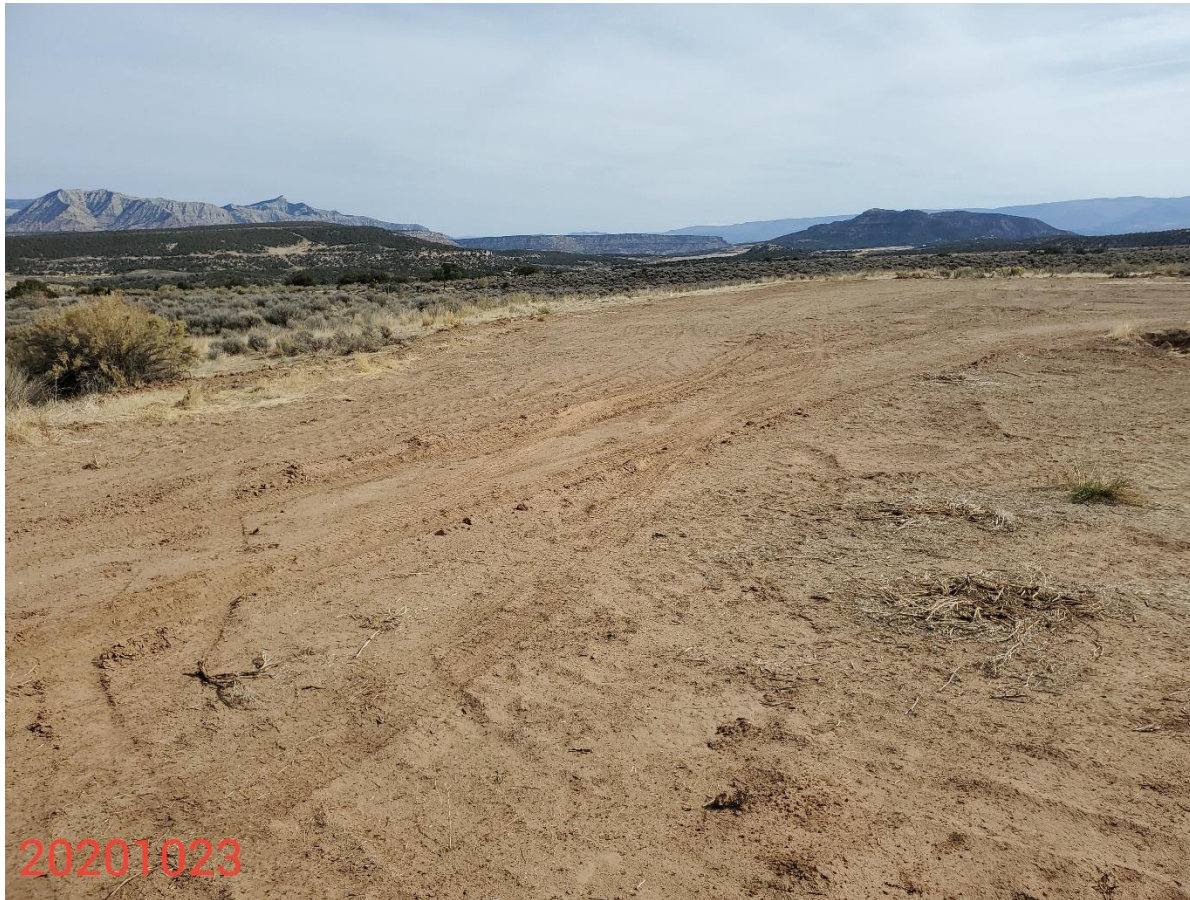
Photo 1: Photo taken from the west end of the location, facing northeast. Photos show surface equipment has been removed from the Location. Location and access road requiring compaction alleviation, contouring/re-grading, replacement of soils and revegetation activities.
