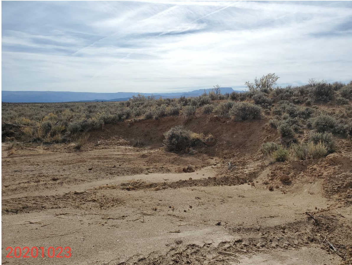
Photo 4: Photo taken from the south end of the Location, facing east. Photo shows cut slopes of the location requiring contour/grading.
