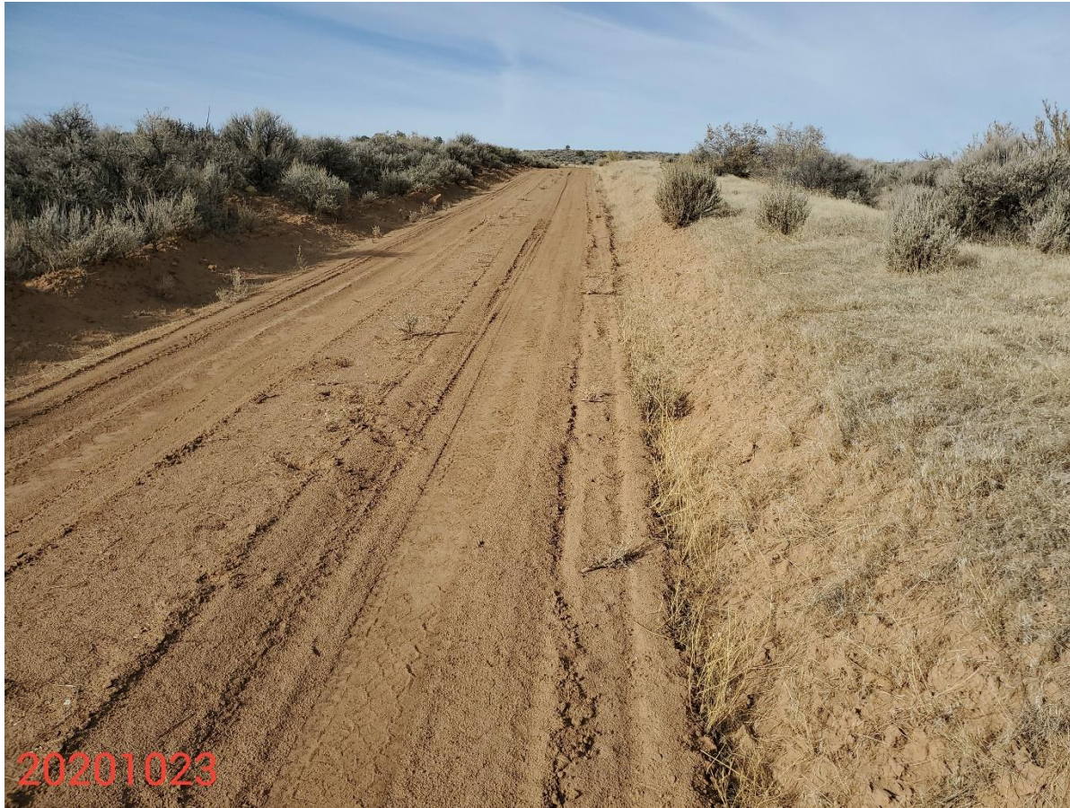
Photo 14: Photo taken from the access road, facing west. Access road requiring compaction alleviation, recontouring/regrading and revegetation activities pursuant to Rule 1004.a.
