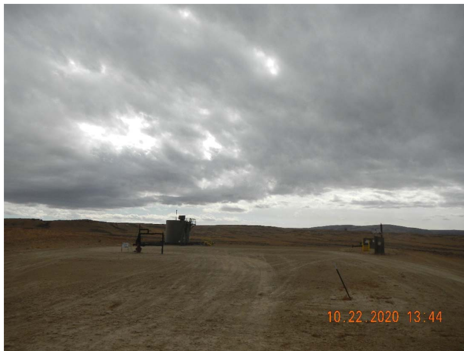
Photo 1. Overview of location taken facing west.
